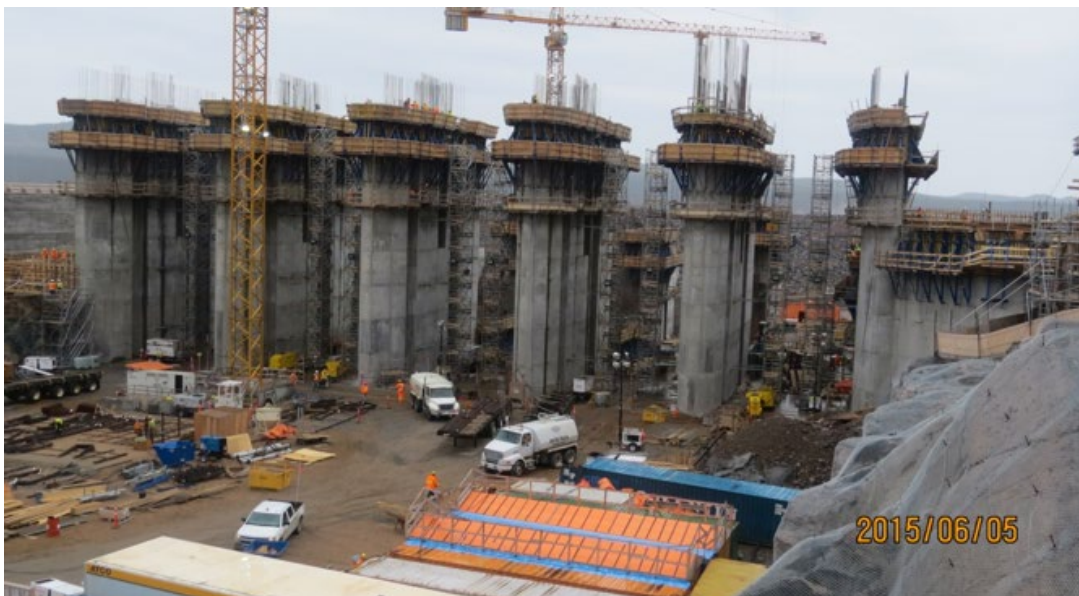
Progress on the Spillway, June 5, 2015
