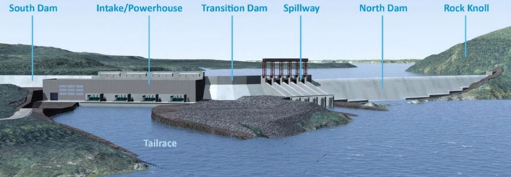
Figure showing the Muskrat Falls Generating Facility
