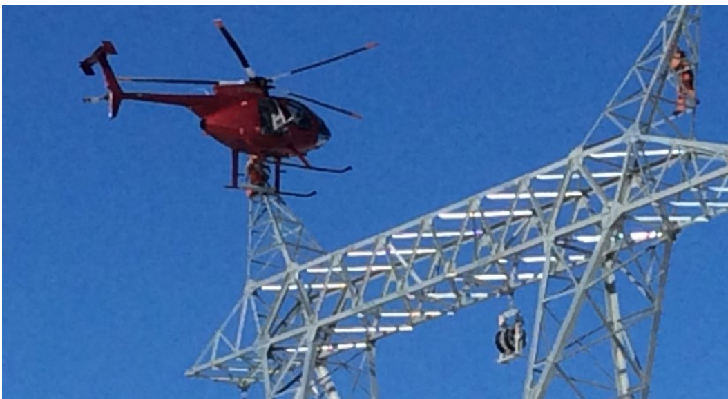
Labrador Transmission Assets Stringing Operations
