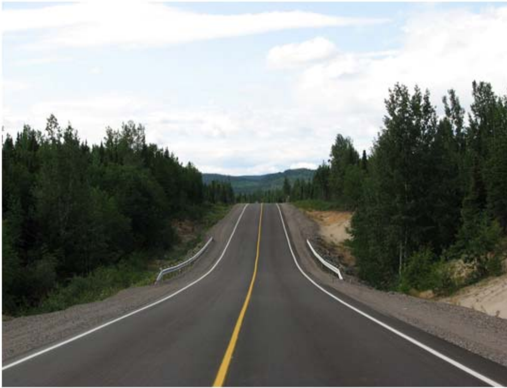
Trans Labrador Highway, Phase I
