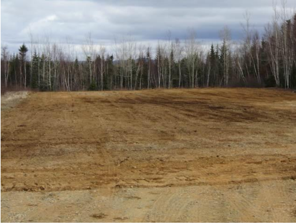
Figure A17. The renovated lingonberry site in Pynn's Brook, ready for prep and planting.
