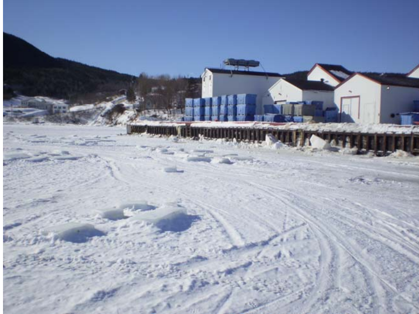
Photo 4.7.2.2 – Photo of marginal wharf taken from harbour
