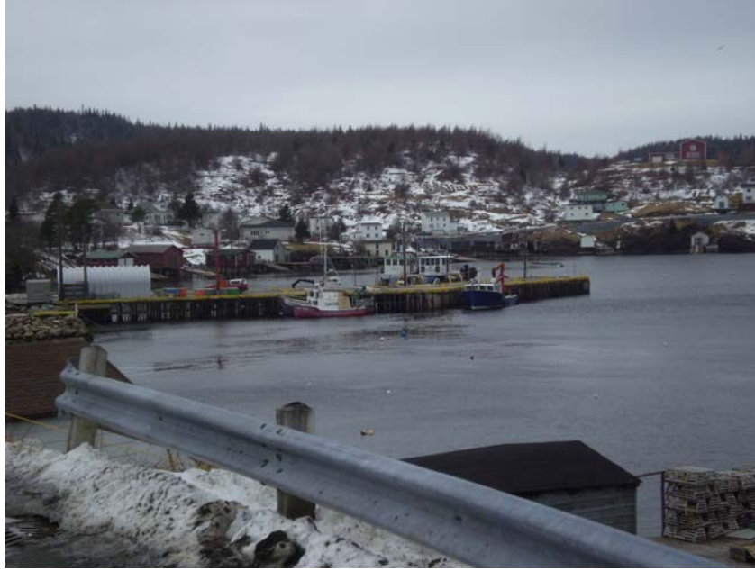
Photo 4.1.2.2 – Photo of wharf looking North
