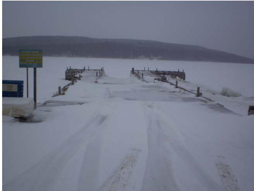
Photo 4.6.2.4 – Photo showing recreation/commercial wharf site
