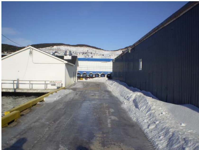
Photo 4.3.2.5 – Photo showing access to wharf #1 from parking area
