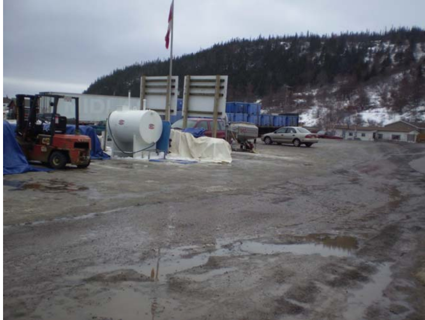
Photo 4.1.2.3 – Existing wharf laydown area
