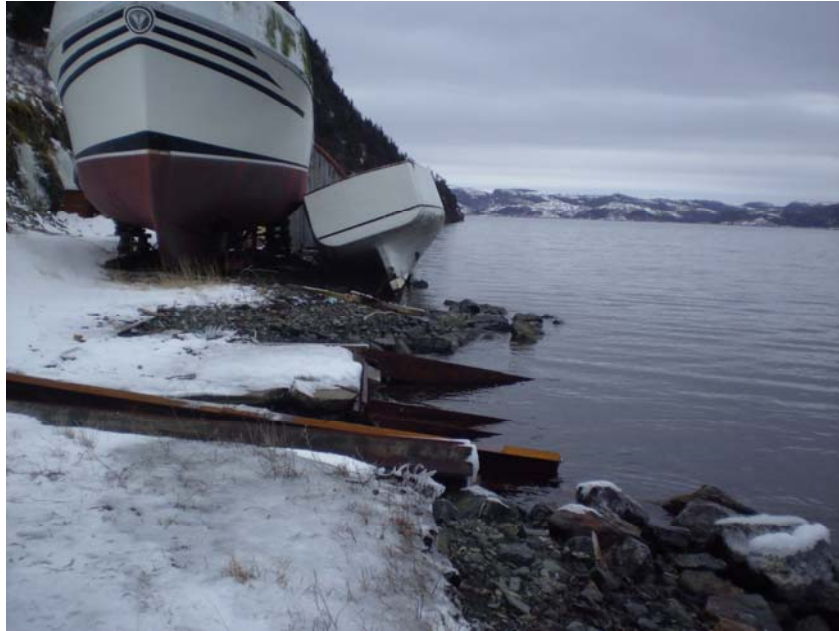
Photo 4.4.4.3 – Photo looking north at possible new outflow wharf site location
