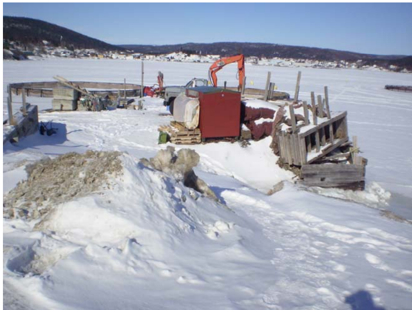
Photo 4.7.2.5 – Nordic Salmon’s private wharf site
