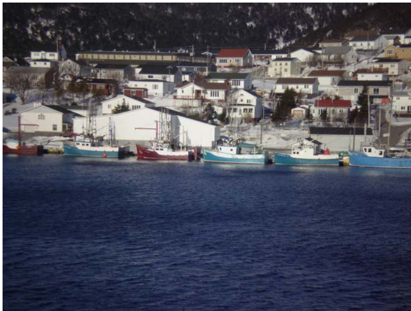
Photo 4.3.2.3 – Photo showing marginal section of wharf #2
