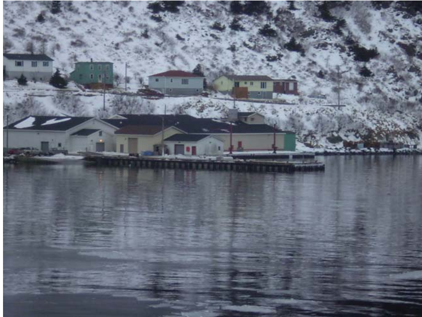
Photo 4.4.2.1 – Photo of ferry wharf finger pier, with fish plant marginal wharf in the right background
