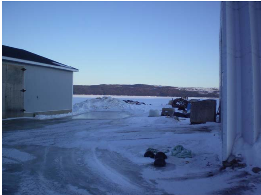
Photo 4.7.2.7 – Photo of Newfoundland Aqua’s existing site
