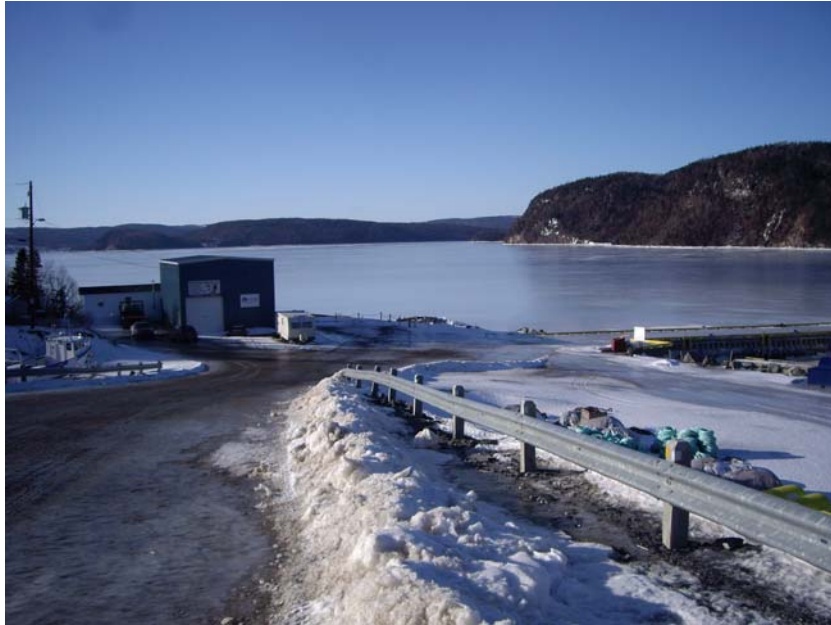
Photo 4.5.2.3 - Band Council bldg. in background with wharf and laydown area to the right
