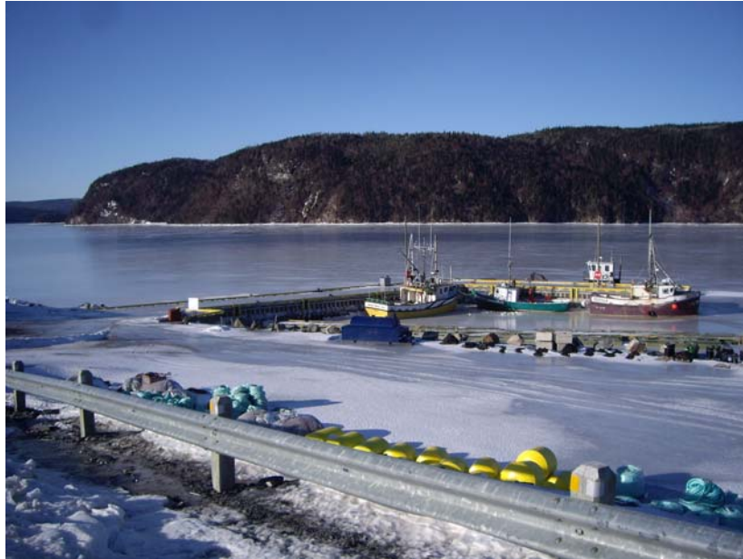
Photo 4.5.2.1 – Photo of wharf looking west toward the harbour entrance
