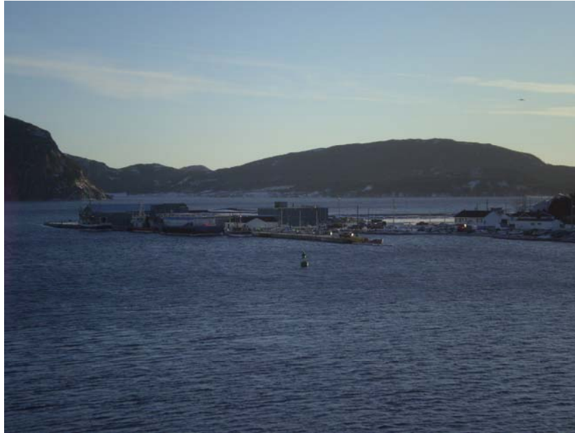
Photo 4.3.2.1 – Photo looking at wharf #1, with fish plant visible in the left background
