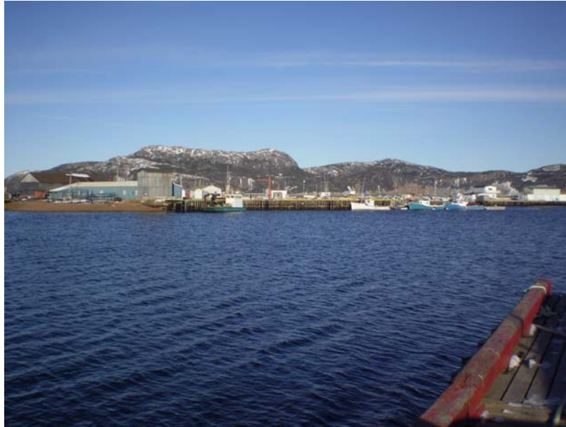
Photo 4.2.2.1 – Photo of public wharf taken from the former Coastal Boat Wharf with fish plant visible in left background
