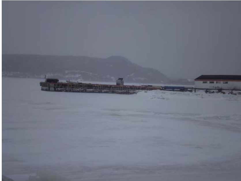
Photo 4.6.2.1 – Photo of leeward side of wharf showing approach and storage shed to the right
