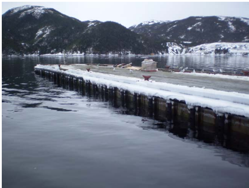
Photo 4.4.2.2 – Photo of ferry wharf looking out from the fish plant wharf
