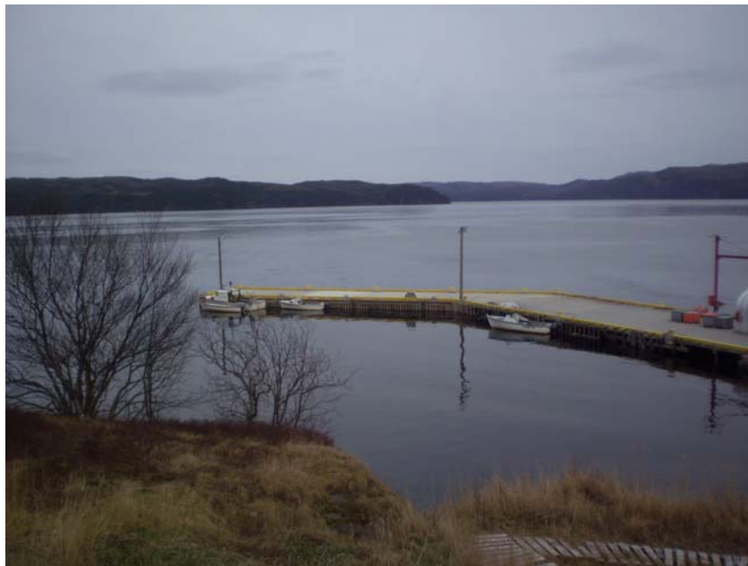
Photo 4.1.2.1 – Photo of wharf looking east toward harbour entrance
