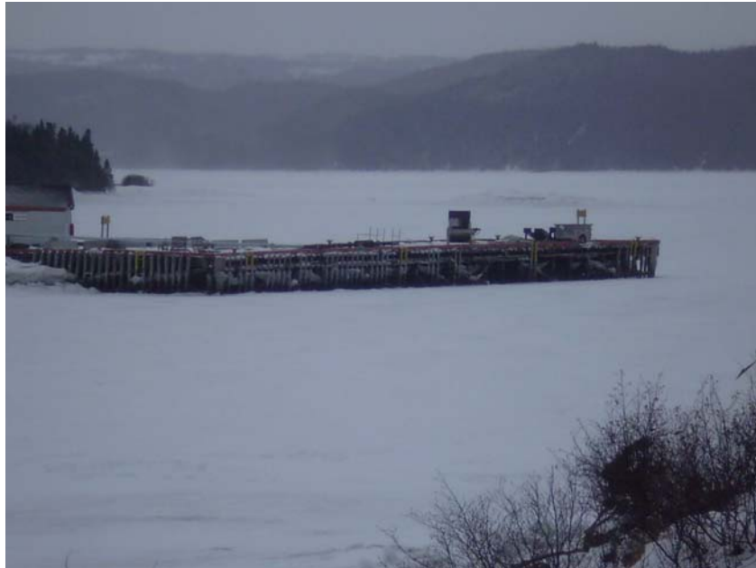
Photo 4.6.2.2 – Photo of wharf showing seaward side
