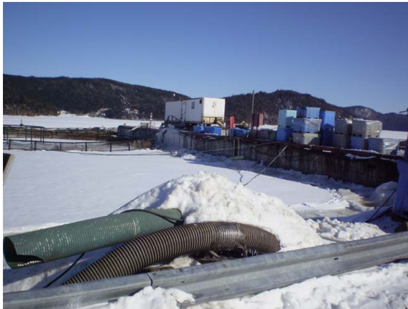
Photo 4.7.2.1 – Photo of finger pier looking from access road
