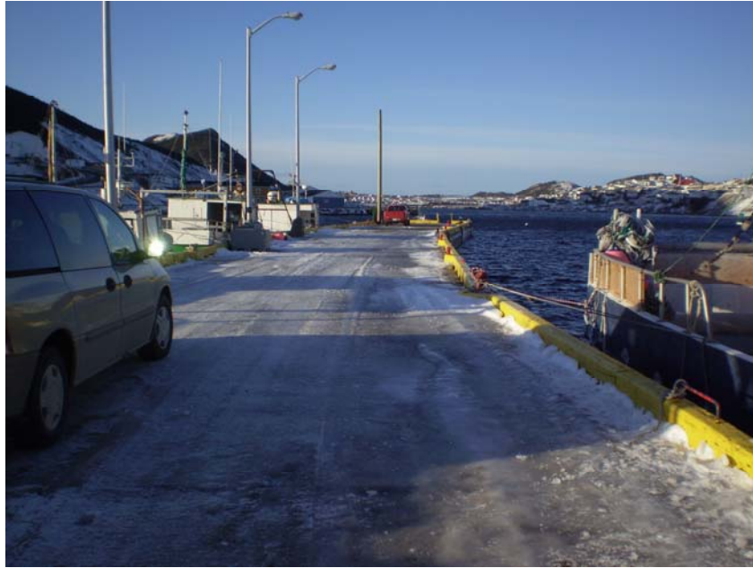
Photo 4.3.2.2 – Photo showing finger pier section of wharf #1
