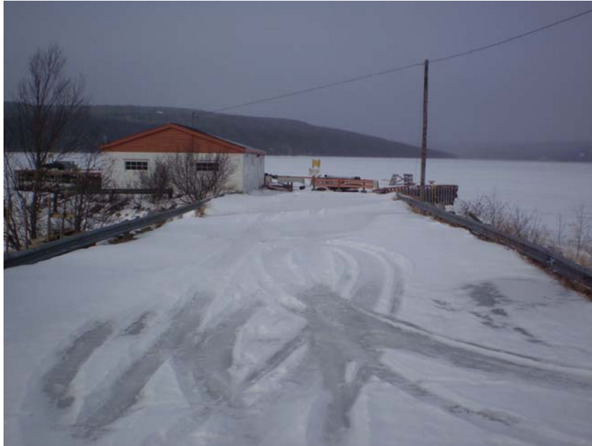
Photo 4.6.4.1 – Photo looking at existing structure and possible new inflow site location
