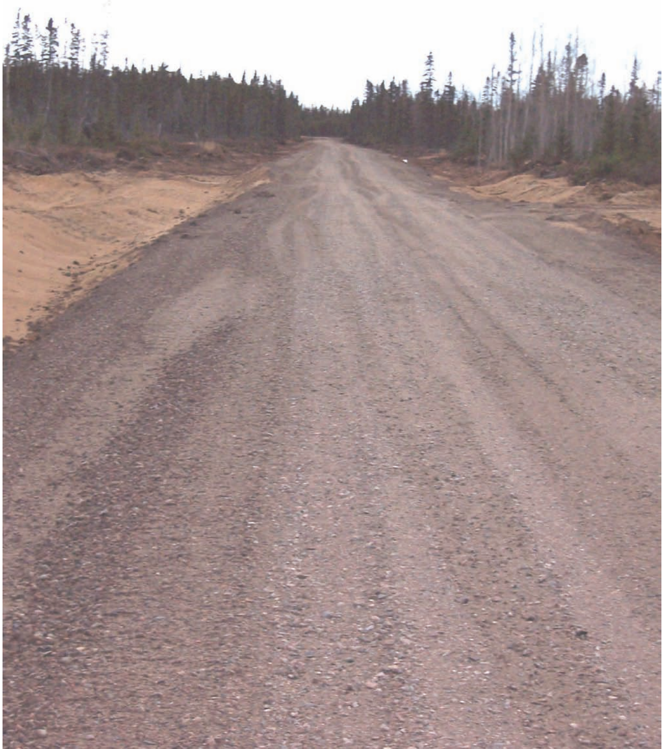
ACCESS ROAD LOOKING NORTH
