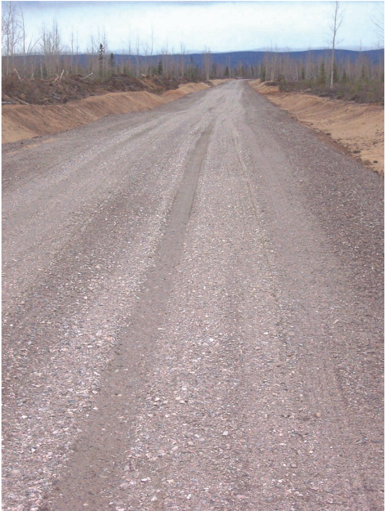
ACCESS ROAD LOOKING TOWARD CHURCHILL RIVER
