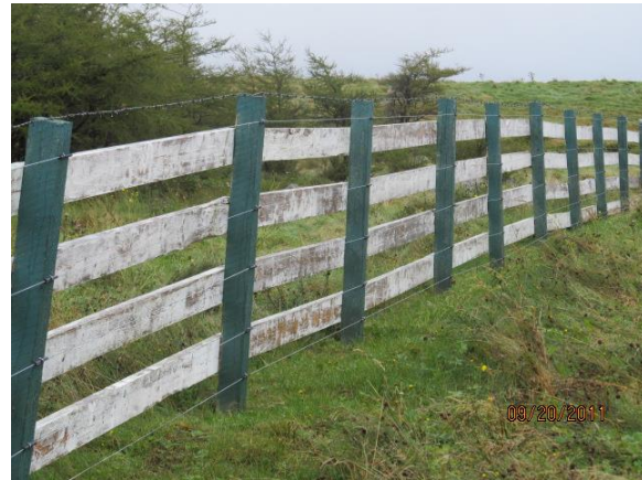
Figure 3. The 5-strand electric fencing and block wire fencing installed at Long Harbour Pasture.
