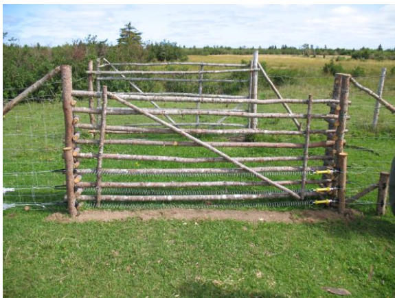
Figure 2. The 3-strand electric fencing and page wire fencing installed at Port-au-Port Pasture.
