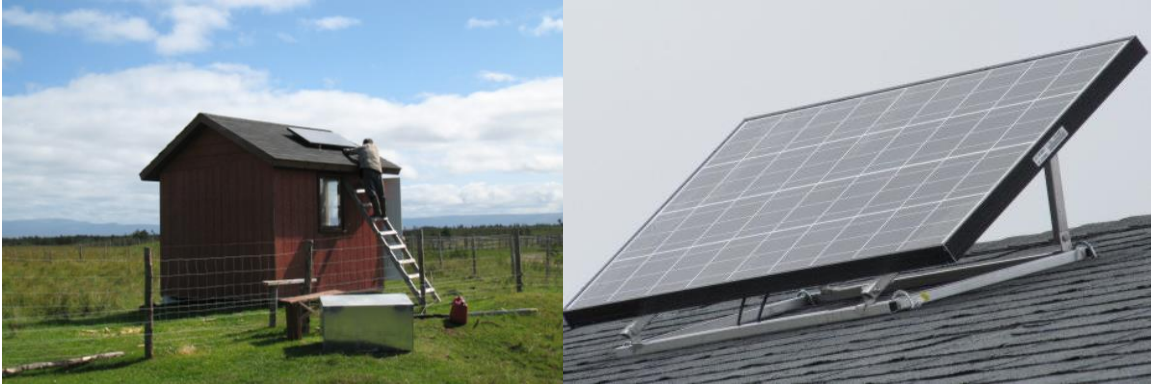
Figure 5. Solar panel power sources on the top of the pasture buildings at Port-au-Port and Long Harbour Pastures.
