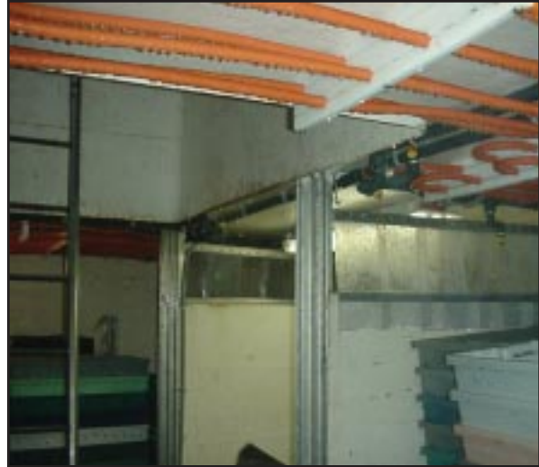
Fresh seawater surges through the system.
