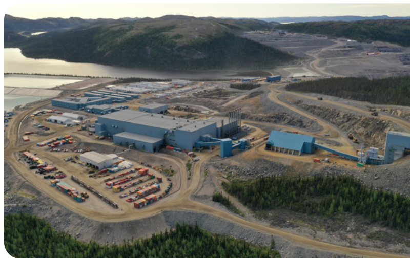
Vale's Open-Pit Mine and Concentrator at Voisey's Bay Photo courtesy of Department of Industry, Energy and Technology
