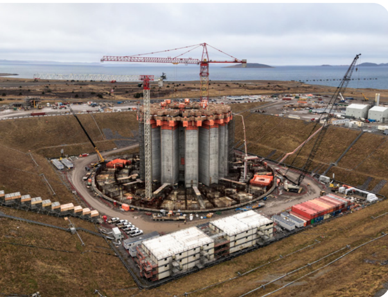
West White Rose Extension Concrete Gravity Structure
