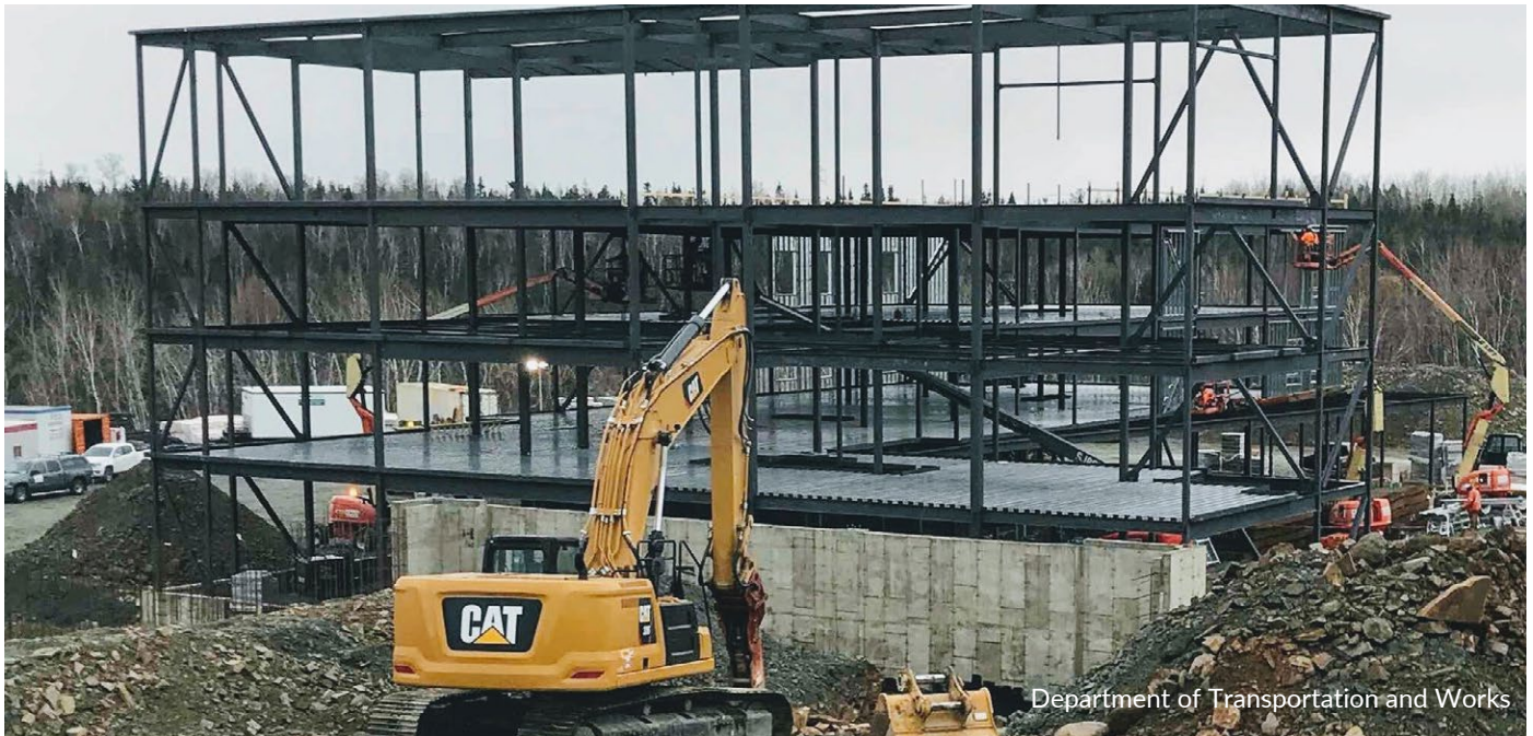
Construction of Long-Term Care Home in Grand Falls-Windsor
