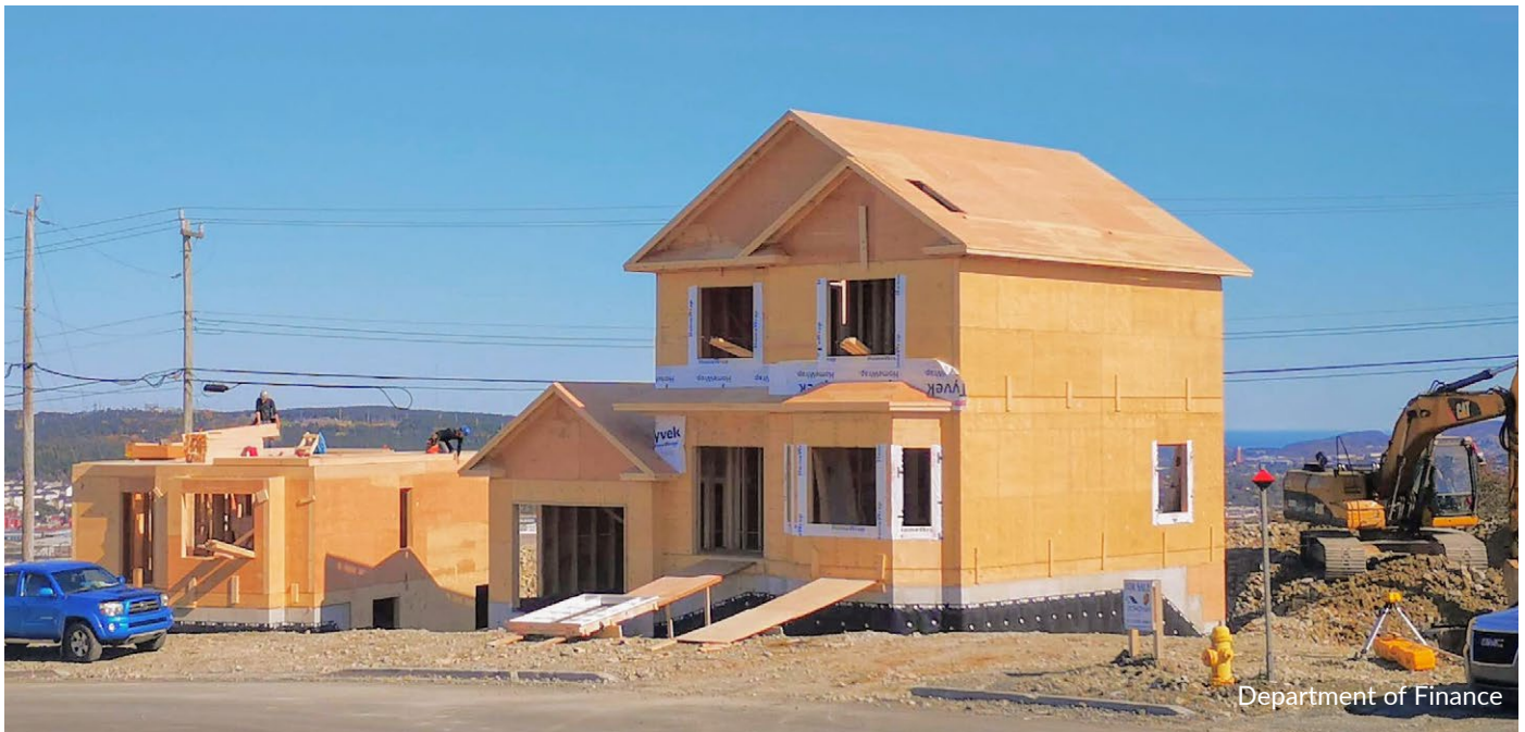
New Home Construction, St. John's
