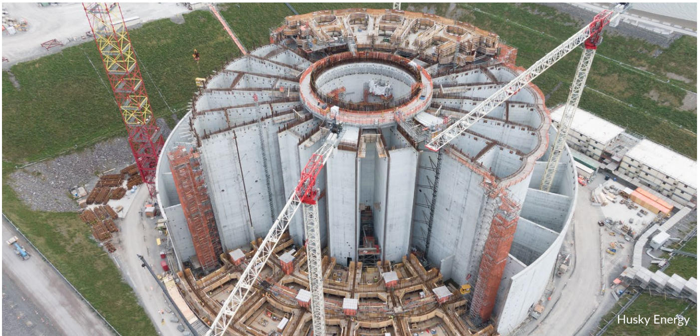
West White Rose – Construction of Concrete Gravity Structure in Argentina
