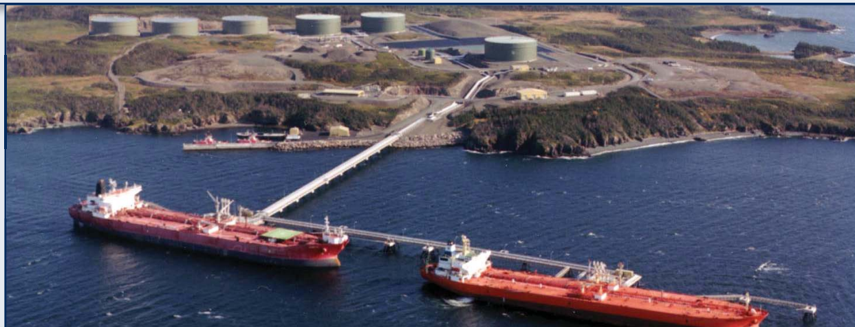
Vessels offloading crude oil at the Newfoundland Trans-shipment Terminal, Whiffen Head
