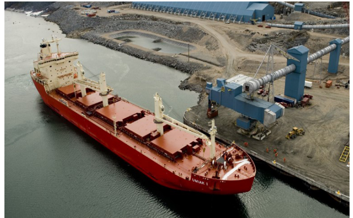
Loading the UMIK 1 at Voisey's Bay Port Site Photo Credit - Vale Newfoundland and Labrador Limited
