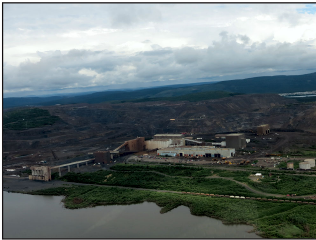
Plate 4. Aerial view of Wabush Mines concentrator, with Scully Mine in background.
