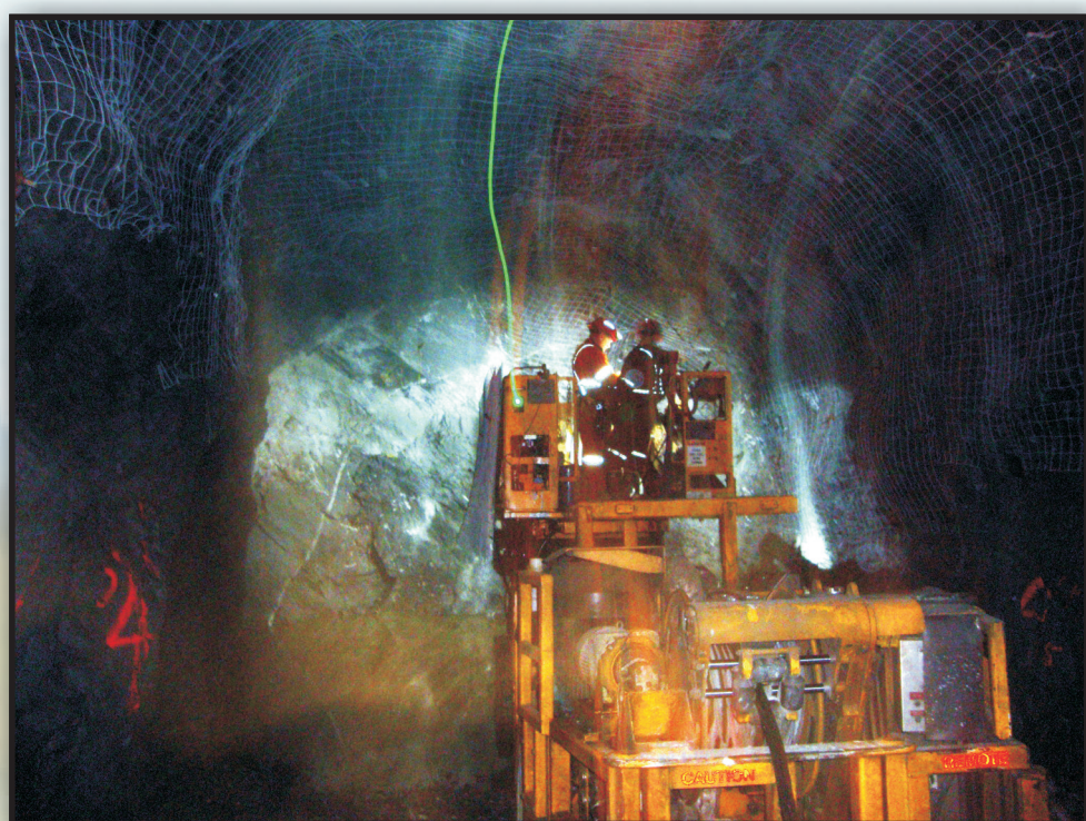
Ground support crew at level 460 installing rock bolts
