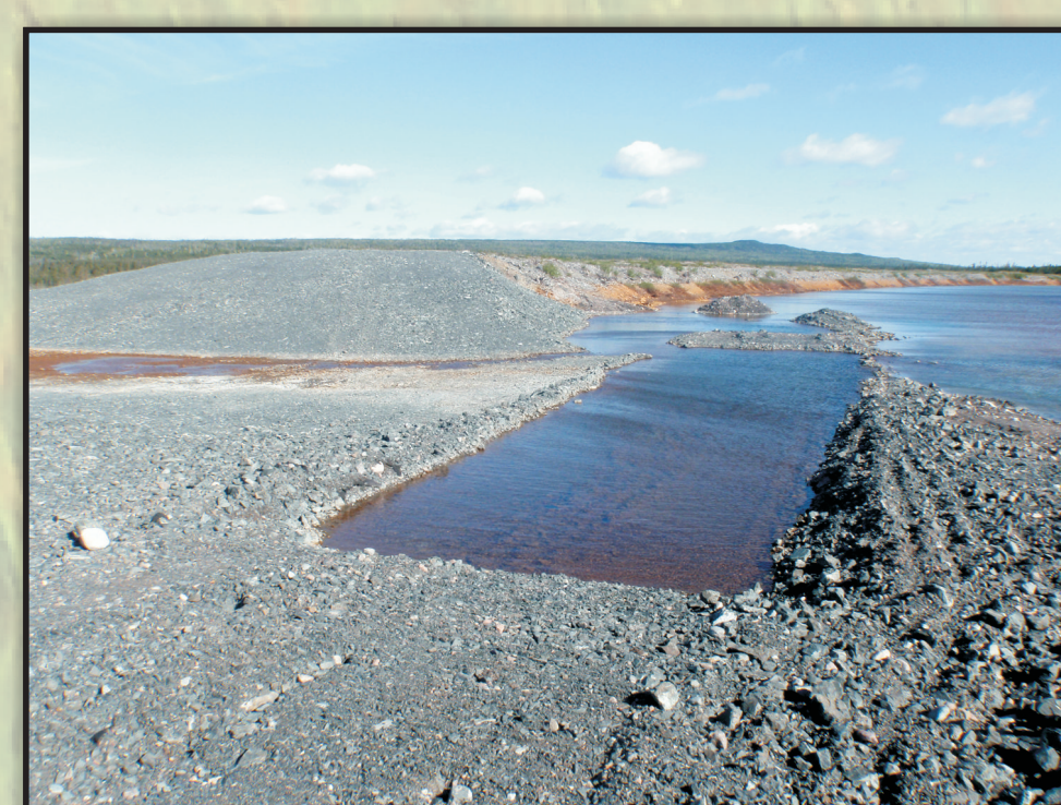
Gullbridge breach after repair
