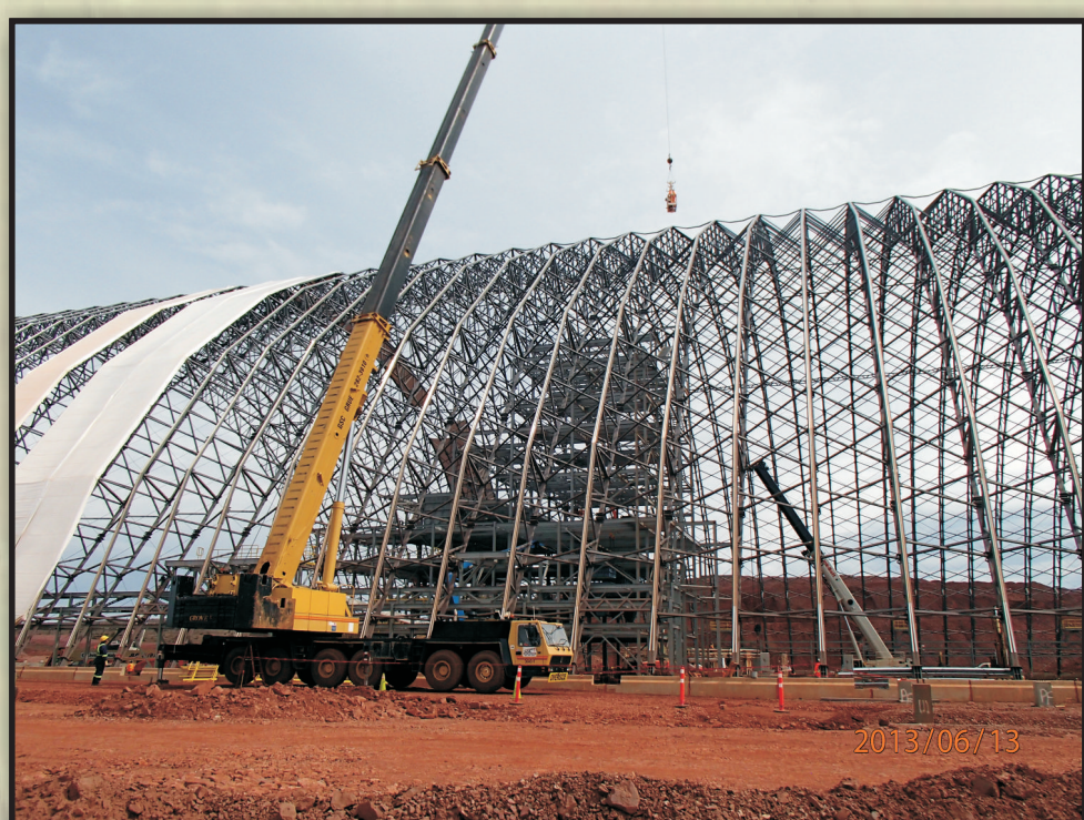
Covering the dome structure
