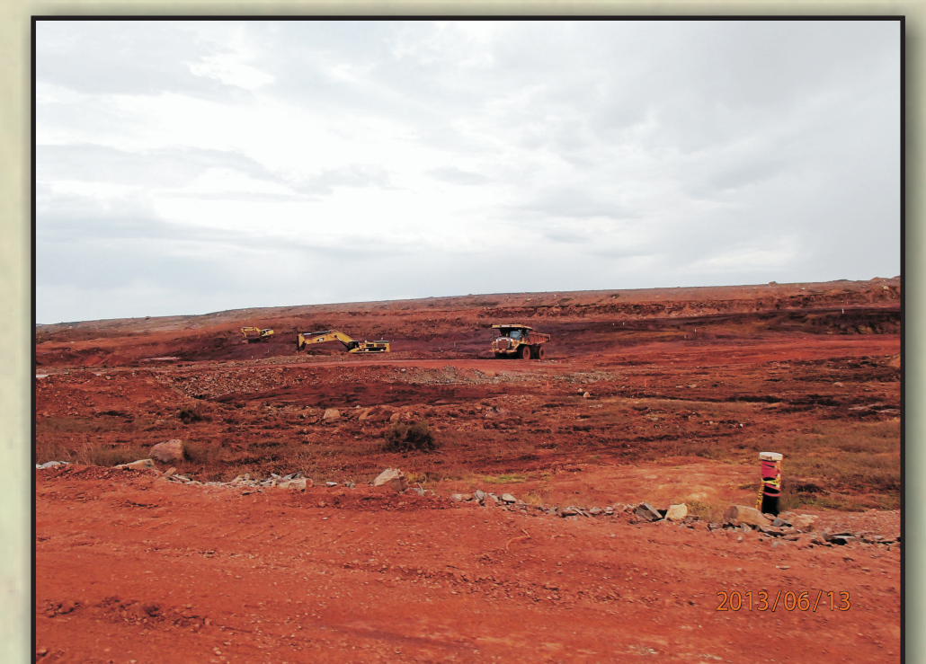
Fleming 7N - Overburden stripping
