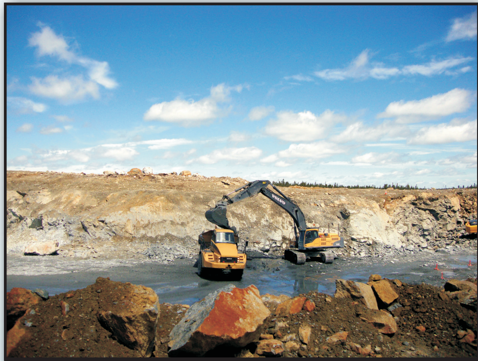
Boundary deposit North-pit (Ore mucking after the bench blast)
