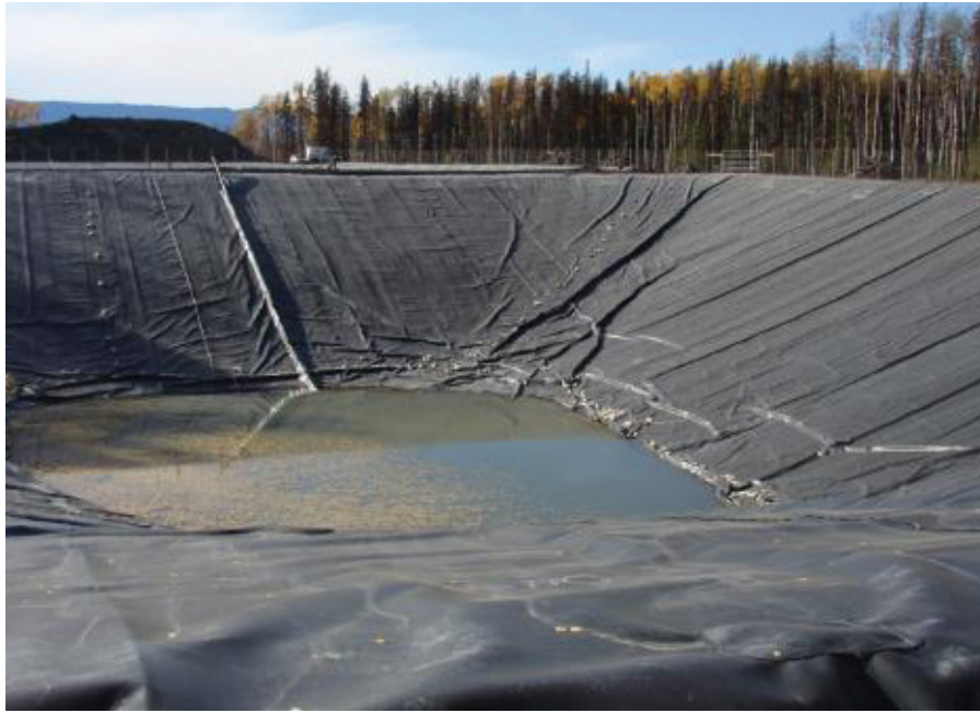
Figure 5.5.13. Liner in an evaporation pond.
