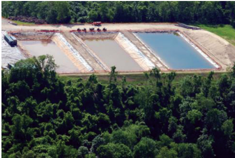
Figure 5.5.12. Evaporation ponds storing flowback and produced water.
