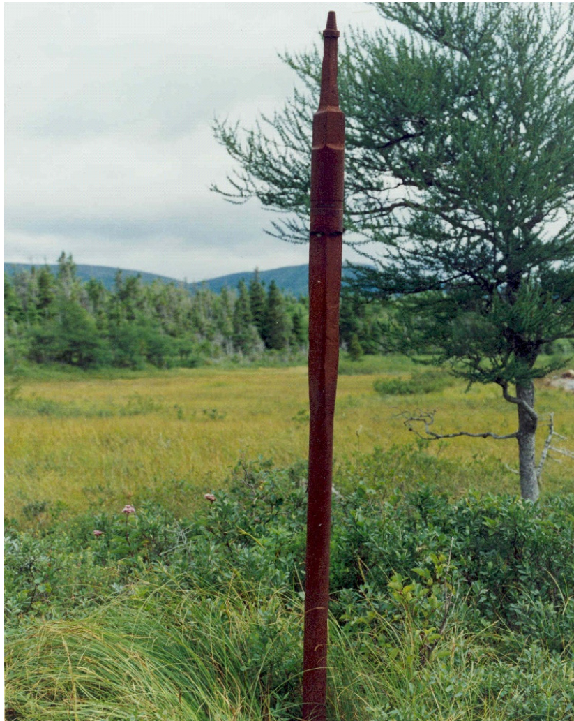
Figure 39. An abandoned legacy well from the Parsons Pond area. In the early part of the 20th century the drill stem became trapped in the hole. Photo courtesy of L. Hicks.
