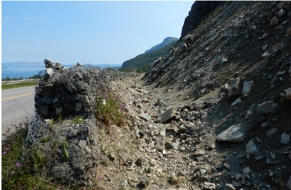
Figure 14. Stone and wire mesh barrier near York Harbour is damaged from falling debris and including with boulders that leap this barrier and cross the highway.
