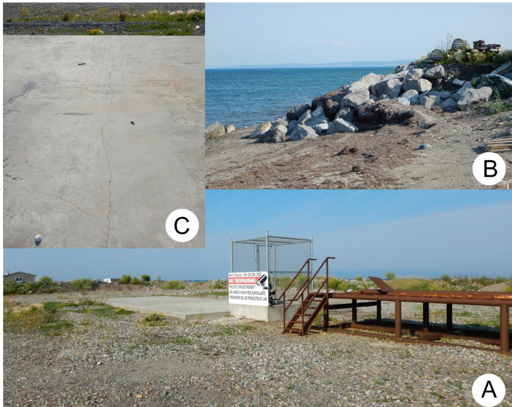
Figure 22. Shoal Point K-39 well site at the tip of Shoal Point in Port au Port Bay (A) with a berm surrounding the site and covered with boulder rip-rap (B). The thick concrete pad adjacent to the north side of the fenced well head is cracked (C).
