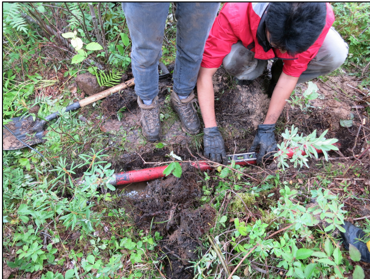
Placing a coil underground
