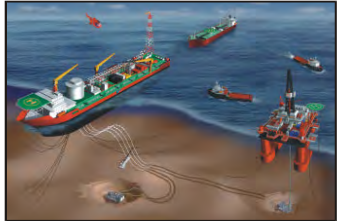
Terra Nova Floating Production Storage and Offloading Facility
