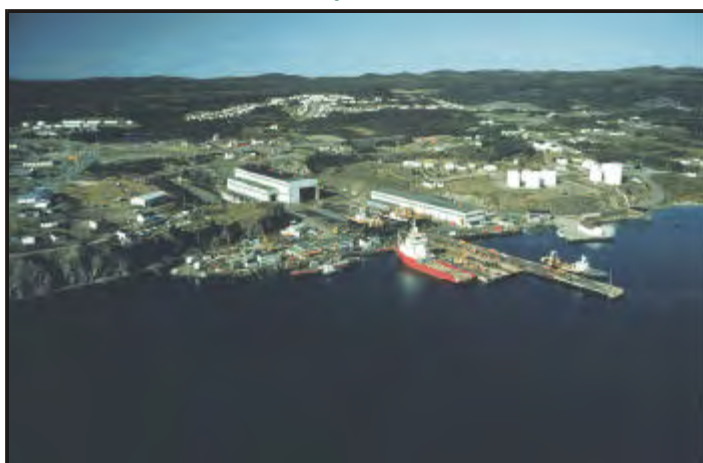
Figure 2.8 Friede Goldman Facility at Marystown
