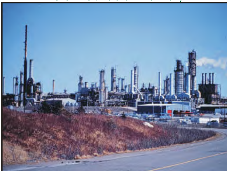
Figure 2.7 North Atlantic Oil Refinery
