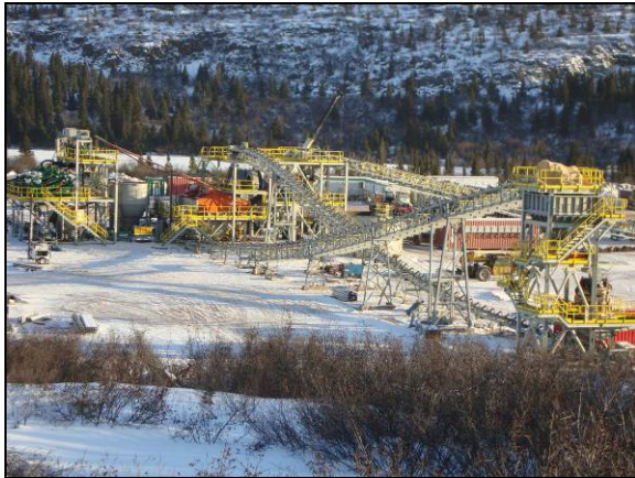
Schefferville Project - Labrador Iron Mines
