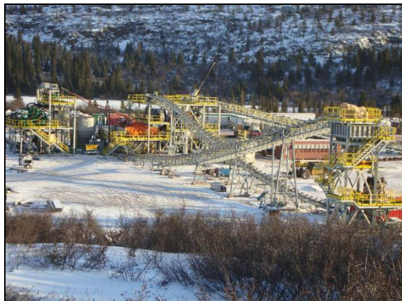
Plant construction – Schefferville Project, Labrador Iron Mines
