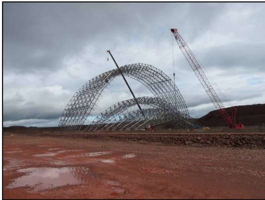
Dome construction – DSO Project, Tata Steel Minerals Canada Ltd.
