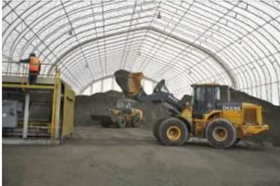
Concentrate Storage Shed, Rambler Metals and Mining PLC
