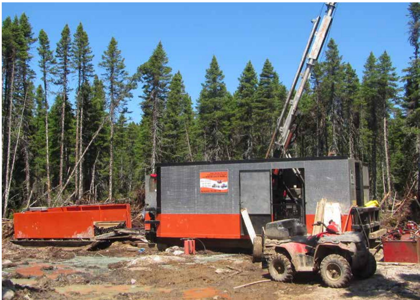
Drill rig, South Tally Pond zinc-lead-copper-silver-gold project, Canadian Zinc Corp.
