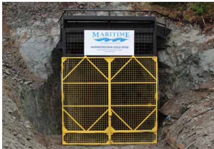
Re-opened mine portal, Hammerdown gold project, Maritime Resources Corp
