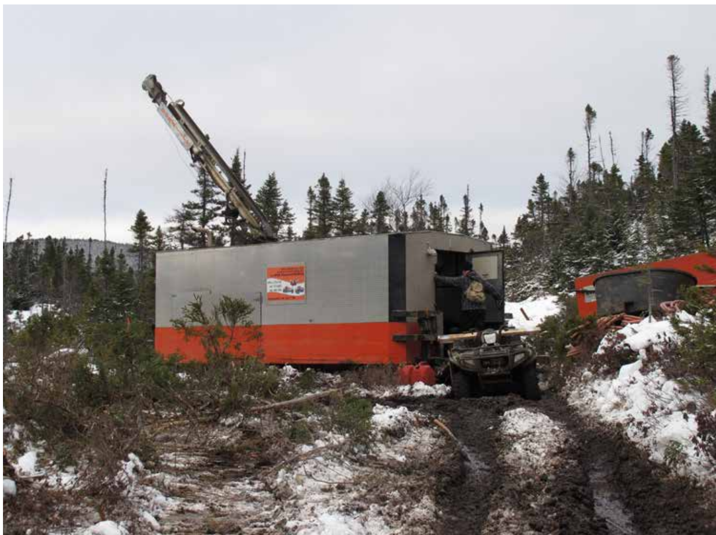
Drill rig, Colchester gold project, Vulcan Minerals Inc.
