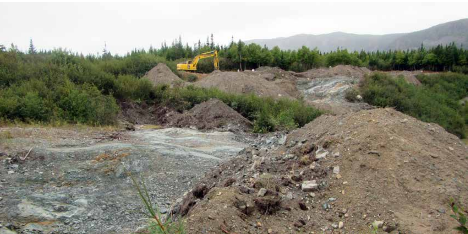
Trenching, Hammerdown gold project, Maritime Resources Corp.
