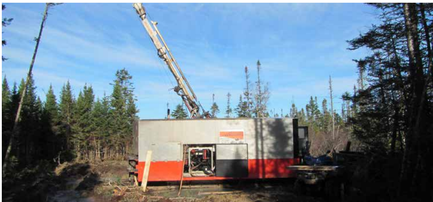
Drill rig, South Tally Pond zinc-lead-copper-silver-gold project, Canadian Zinc Corp.
