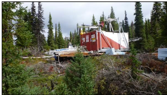
Drilling on the Michelin uranium project, Aurora Energy Ltd.
