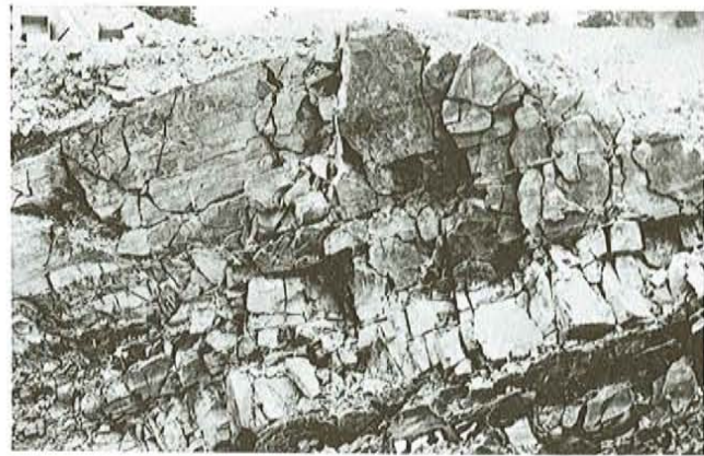
Plate 4. Numerous fractures in a road-cut.
