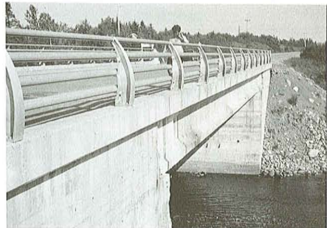
Plate 8. Bridge in excellent condition, no cracking or weathering observed.
