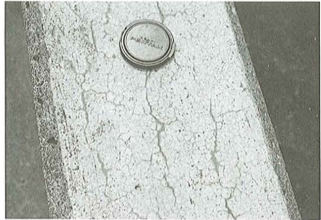
Plate 14. Dry shrinkage cracks in concrete bridge railing.
