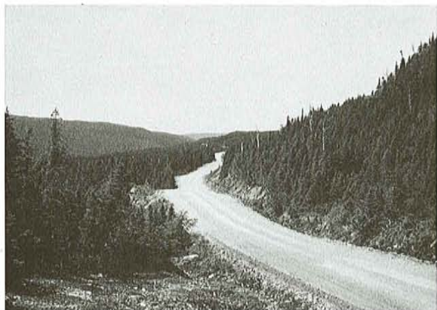
Plate 2. Upgraded gravel road, which branches westward from paved route 420, has greatly improved access to the Upper Humber River region.
