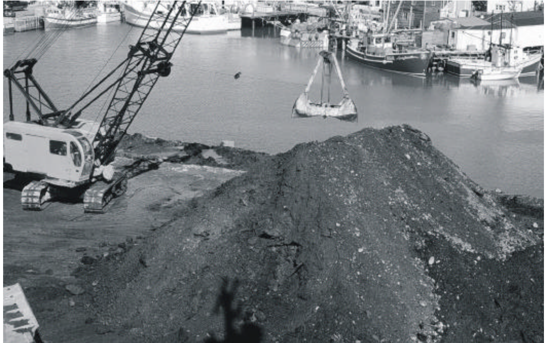
Plate 5. Dredged spoil, Port de Grave, May 1999. Large stumps and fragments of trees are visible on the surface of the spoil pile.
