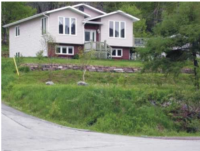
Plate 12b. Garden wall in Woodstock constructed from blocks of the Dunamagon Granite.
