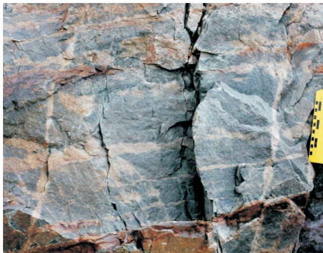
Plate 3. Typical Cape Bonavista facies having a mottled texture, following relatively high permeability corridors along existing fracture systems and subtle variations, located near Bonavista, Bonavista Bay.
