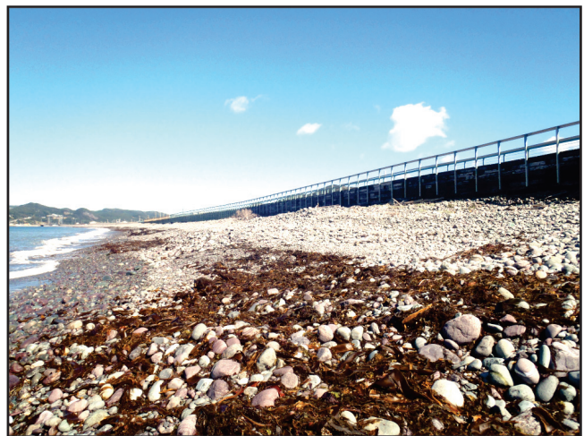
Plate 6: A sea-wall was built along Placentia to provide flood protection. The community of Placentia is built close to sea level on a beach-ridge system, and parts of the community are at risk of flooding due to waves, high tides and storm surges.
