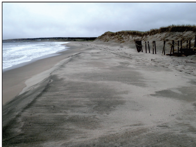
Plate 8. Sand dune at J.T. Cheeseman Provincial Park. The seaward edge of the sand dune eroded 922 cm between 2013 and 2014, exposing an old section of railway.
