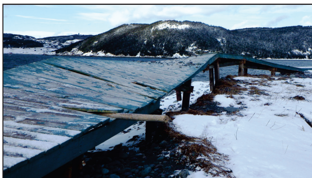
Plate 1. The modern beach in Placentia is a 1.2-km-long pebble-cobble beach. There is a long history of flooding in Placentia, with the area directly landward of the beach at risk from inland flooding and from water overwashing the beach during storm surges and high tides (Liverman et al., 1994). In December 2013 large waves associated with a storm surge caused significant damage to the boardwalk and Beach Road was flooded.
