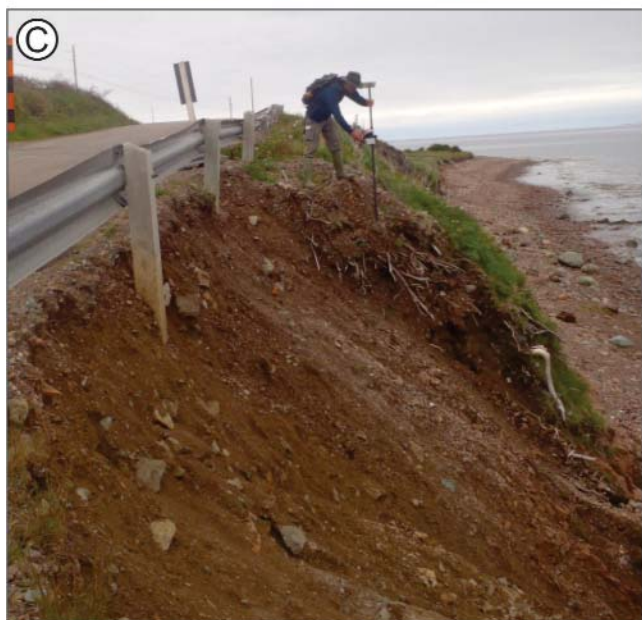
Plate 2. A) Erosion of the unconsolidated slope, landward of a new housing development in Conception Bay South on the Avalon Peninsula, resulted in the closure of a walking trail shortly after its construction; B) In the winter of 2017, the peat cliff along Shoal Point, on the Port au Port Peninsula, eroded and a shed fell off the cliff (circled); C) Coastal erosion has threatened a portion of the main road in Grand Beach, Burin Peninsula; D) Erosion of the coastal cliff at Parson's Pond, on the Great Northern Peninsula, is compromising the stability of the gravel parking lot. Large boulders have been placed to discourage access to the cliff edge.
