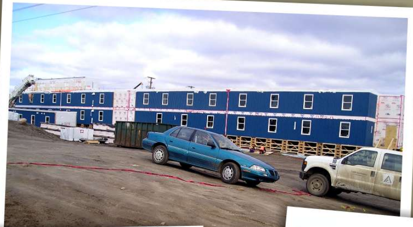
IOC Expansion - Bunk houses under construction
