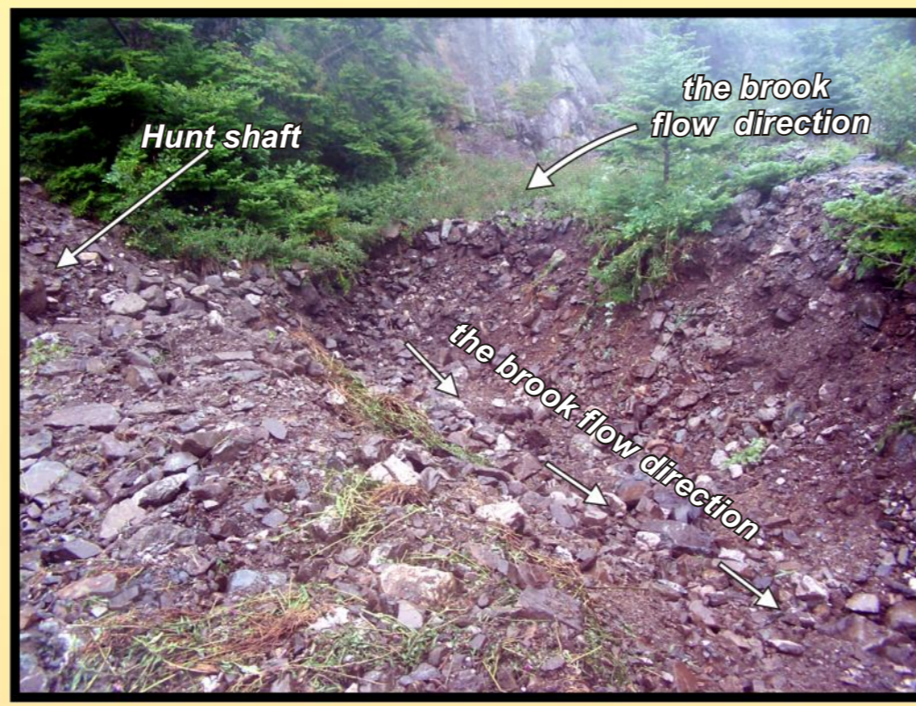
View of excavated ditch around Hunt shaft.
