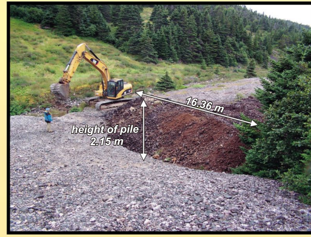
View of Cohu shaft before and after rehabilitation
