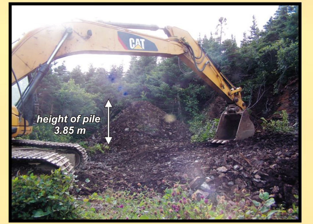
View of McConachie shaft before and after rehabilitation
