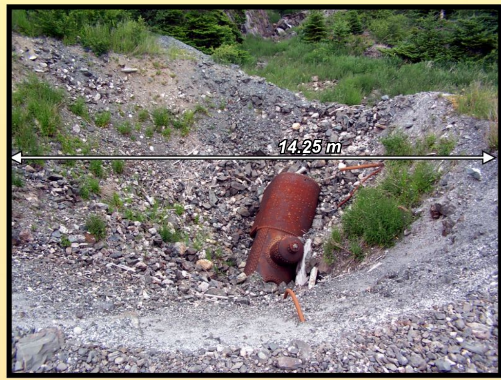
View of Hunt shaft before rehabilitation
