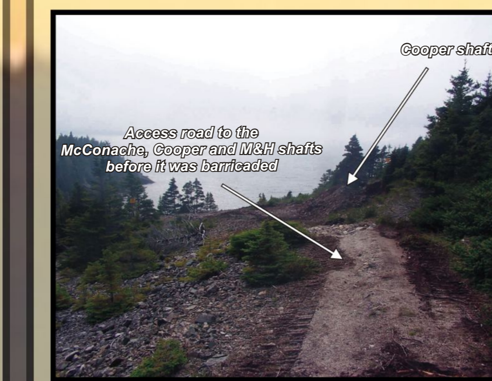
Access road to the McConachie, Cooper and M&H shafts before it was barricaded
