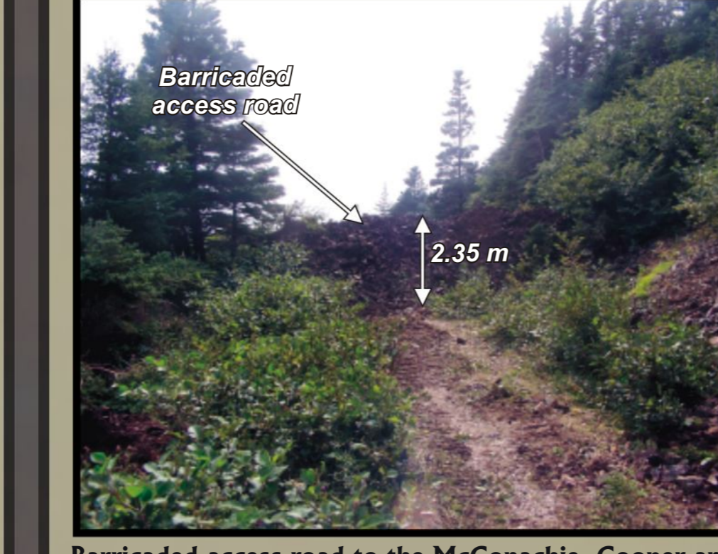
Barricaded access road
