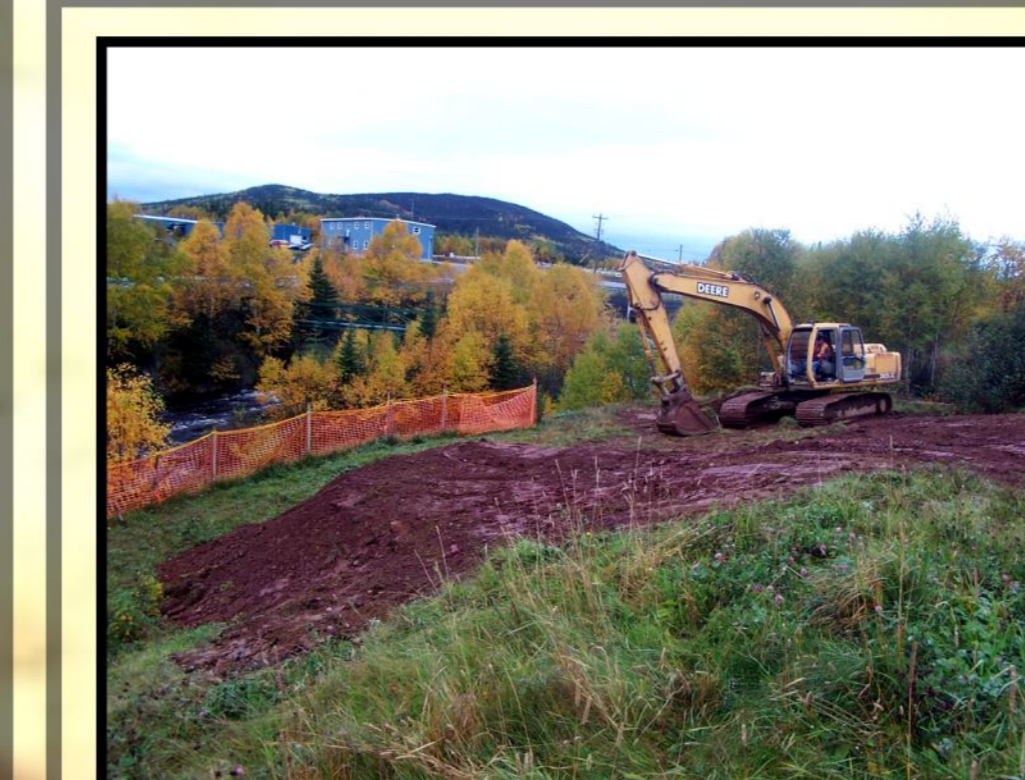
Removed top soil and grass were restored
