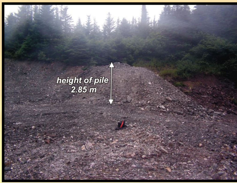
View of Hunt shaft after rehabilitation
