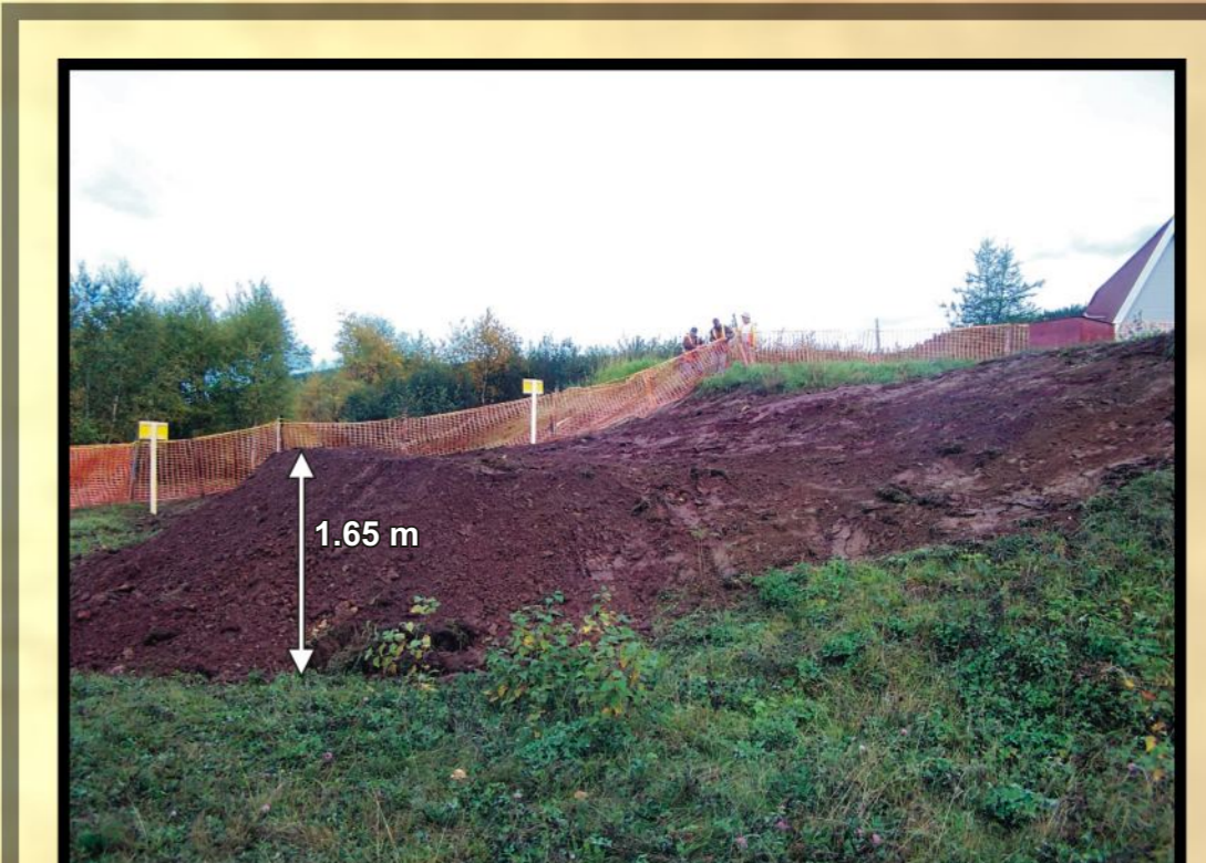
View of the site after rehabilitation completed
