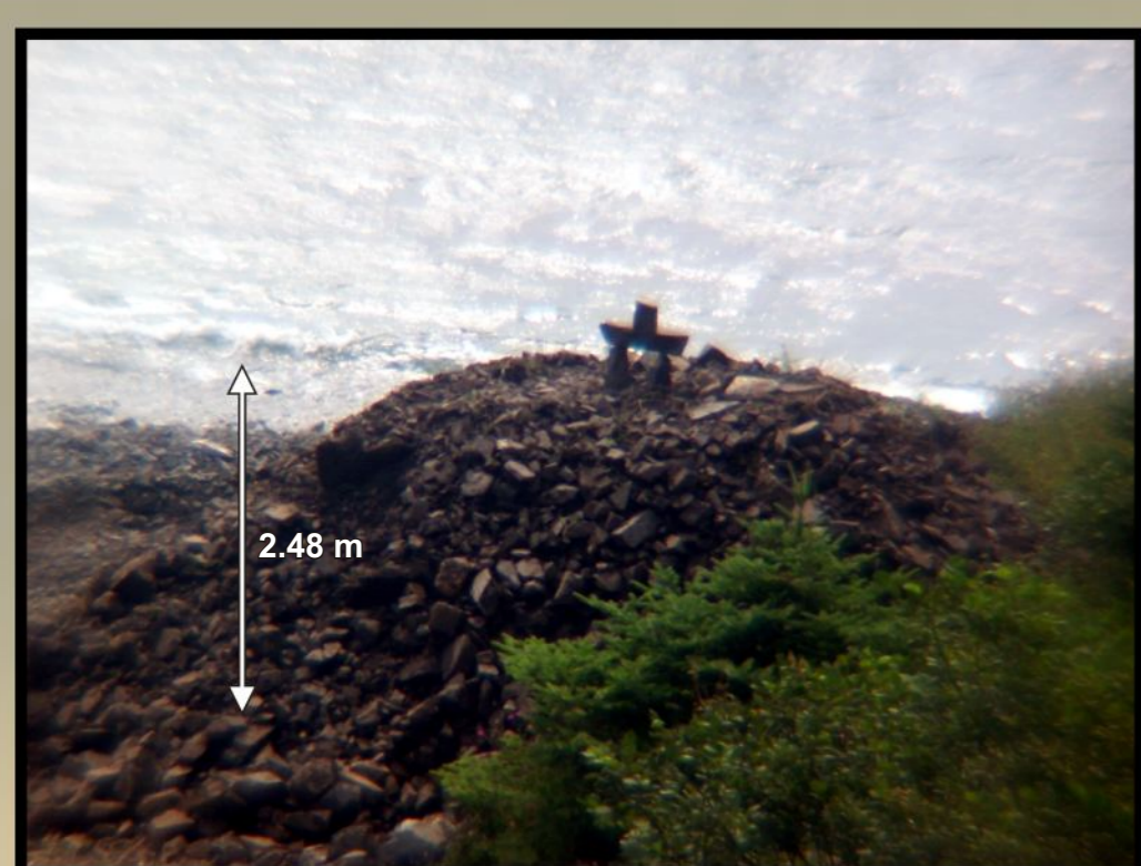
View of M&H shaft after rehabilitation
