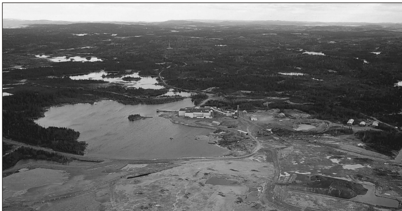
Plate 55. Aerial view (looking east) of the Rambler Mill complex. The small, water-filled pit to the right of the mill is the Footwall Zone open pit. The East Mine headframe is visible in the background.
