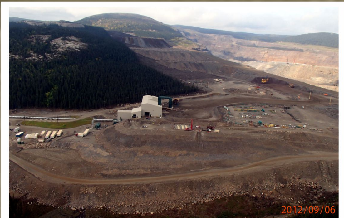
A new crusher and conveyor, the main components of IOC's Concentrate Expansion Program Phase 1, deliver ore from the Luce pit directly to the ore storage barn at the processing complex.
