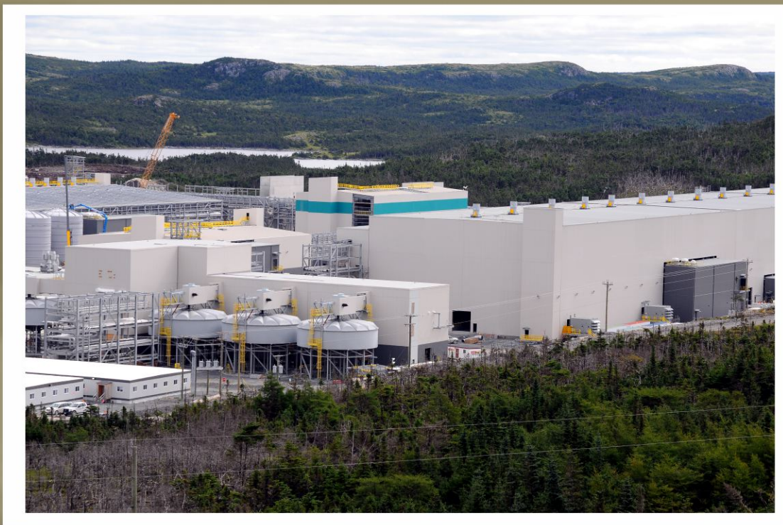
Upper tier, Long Harbour nickel processing plant (Courtesy of Vale Newfoundland and Labrador Limited)
