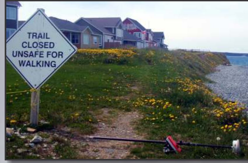
Coastal erosion is occurring in CBS, resulting in the closure of this trail.
