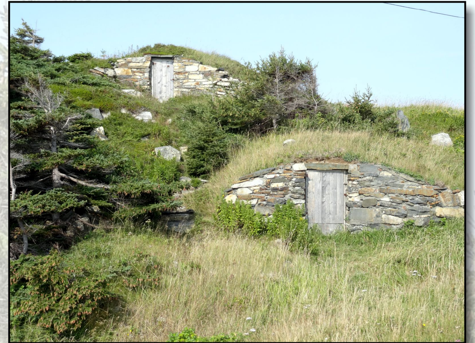
Figure 1. Two root cellars preserved in the town of Elliston, Bonavista Peninsula. Root cellars were built using local flagstone, slate with a well-developed cleavage. This location is a site in the Aspiring Discovery Geopark on the Bonavista Peninsula.
