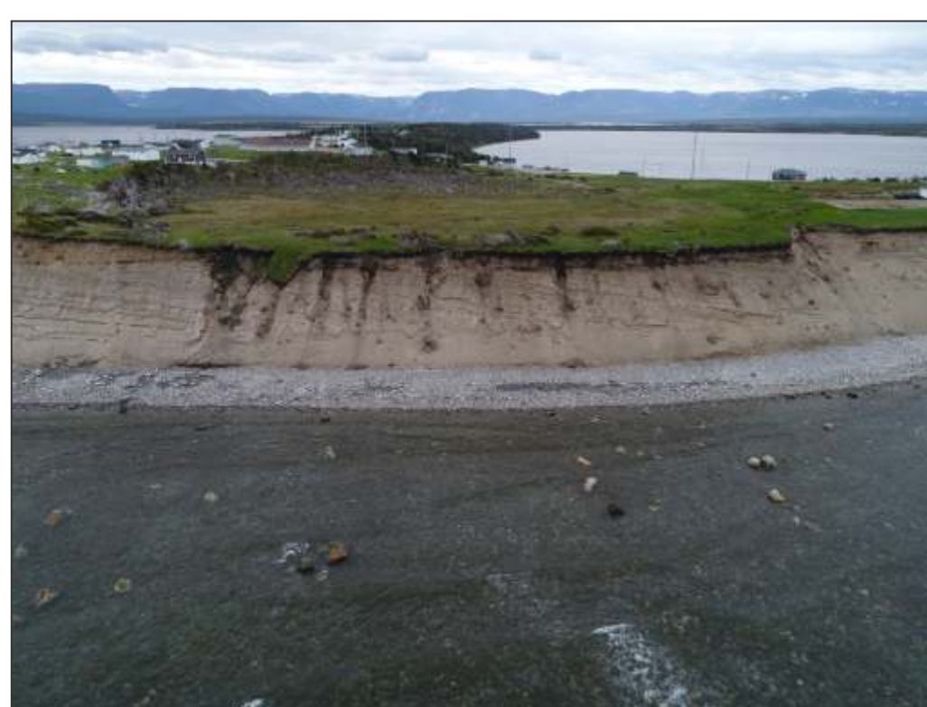
Figure 7: Drone image of coastal cliffs at Parson's Pond, looking east
