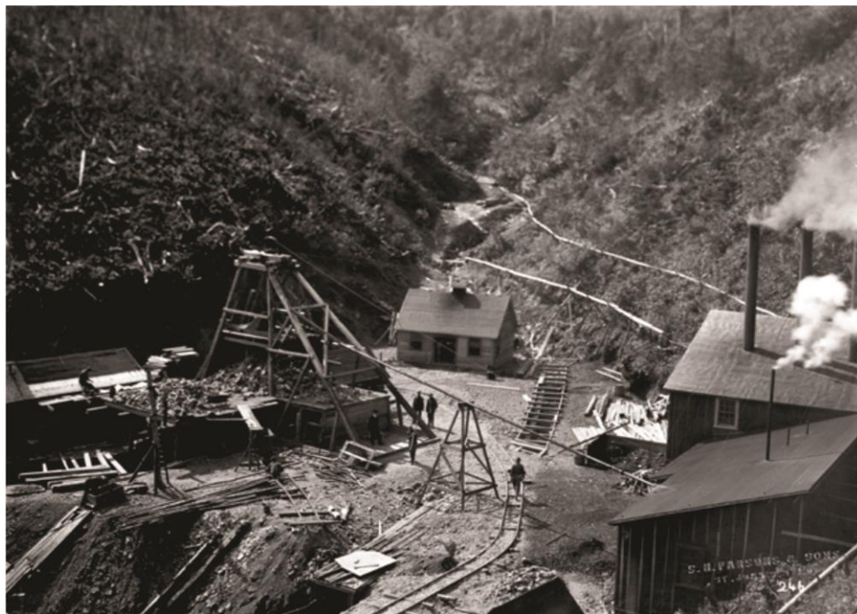
Figure 29: A' Zone shaft and mine buildings, (ca. 1899-1913), York Harbour mine.
