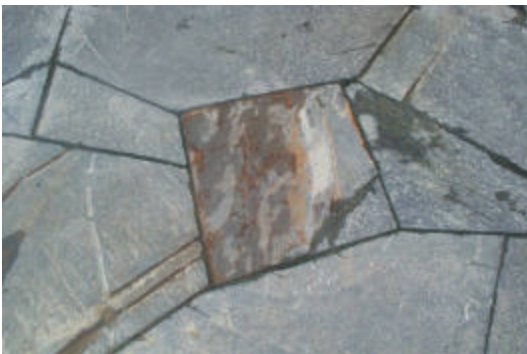
14. Close-up showing detail of stone work
