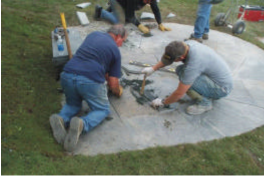
13. Filling seams/joints with sand
