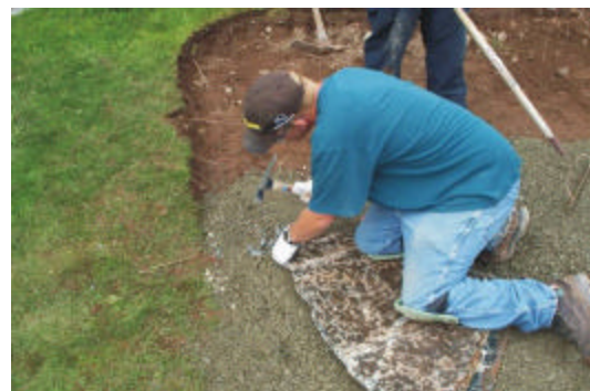
6. Cutting or shaping with a masons hammer
