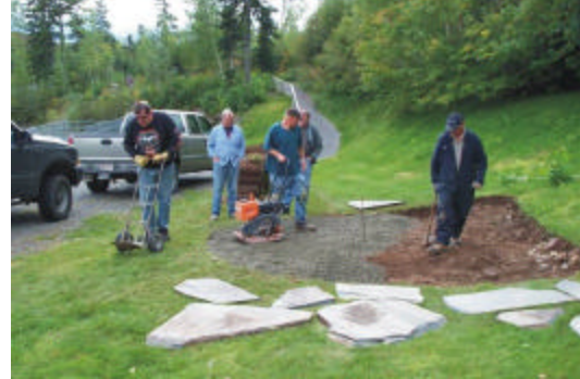
4. Compacting road gravel for base
