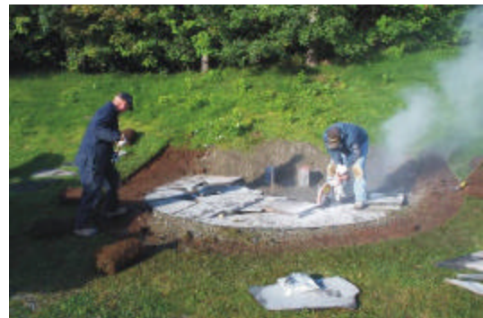
11. Cutting stone with a rock saw
