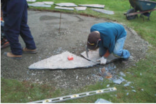
7. Chipping edge to create a tight joint.
