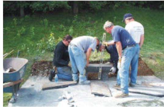
12. Installing the granite bench
