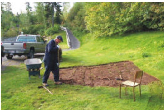
3. Excavating and grading site
