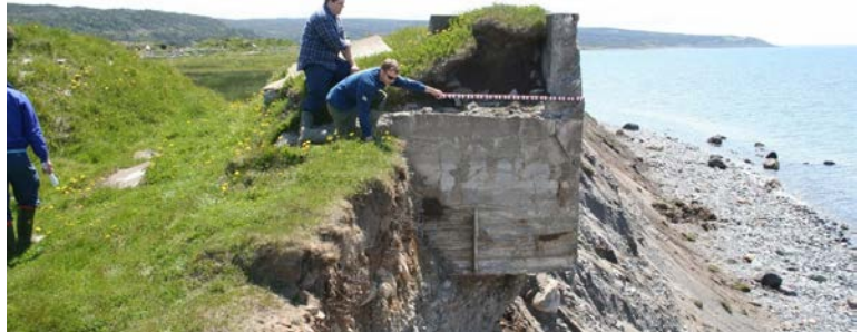
Coastal cliff at Point Verde, 2005. The cliff is eroding at 40 cm/year; wind and water have eroded the sediment under this cement structure which has now fallen to the bottom of the cliff. Quantifying rates of erosion is crucial to determine building setback values to prevent the above loss, as construction impinges on coastal environments.
