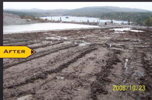
Progressive rehabilitation has commenced. A portion of the area has been backfilled and sloped. Some topsoil replaced and hydro-seeded.
