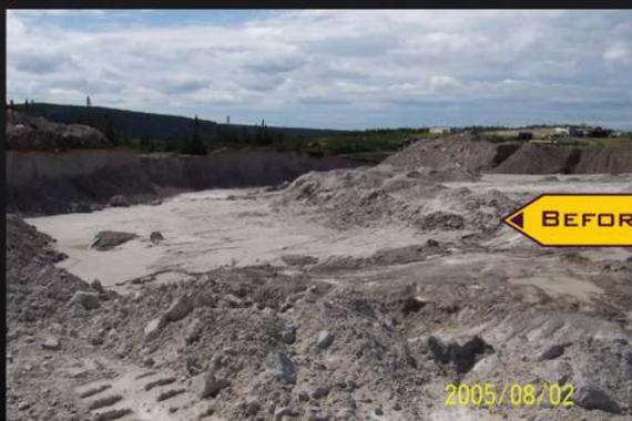
Quarry site has been depleted and rehabilitation has begun. Stage 1 involves backfilling the quarried out area.
