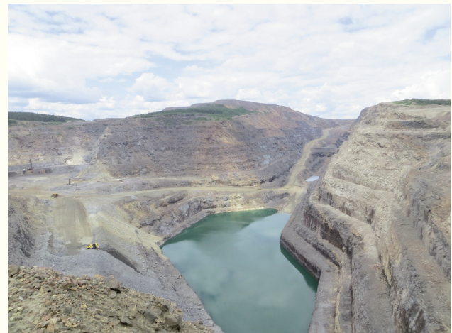
Figure 4. Humphrey Main pit in the IOC’s Carol Lake project.
