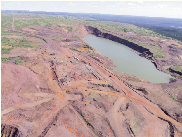
Figure 8. Aerial view of the Timmins No. 1 pit (IOC, exhausted) and construction of Tata Steel Minerals Canada processing facility.
