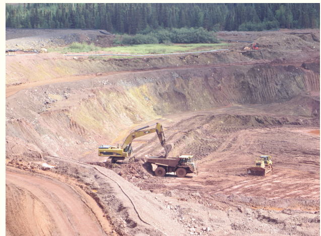
Figure 7. Ongoing excavation at the James Mine (Labrador Iron Mines), Schefferville.
