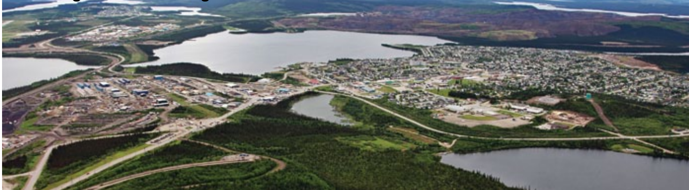
Alderon Iron Ore Corp. is developing the Kami project, located close to the mining towns of Wabush and Labrador City. The project, which is slated for production beginning in Q4 2015, is being developed within a framework of sustainability. Photo courtesy of Alderon Iron Ore Corp.
