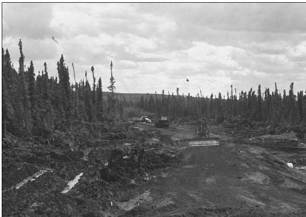
Photo 3: Javelin Road construction summer 1962.
