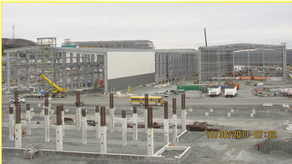
Construction at Vale's Nickel Processing Facility.
