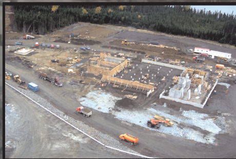
Minesite Construction, Duck Pond
