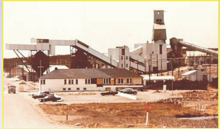
ALCAN Mining Operations, ca. 1977. Surface Works at Director mine.
