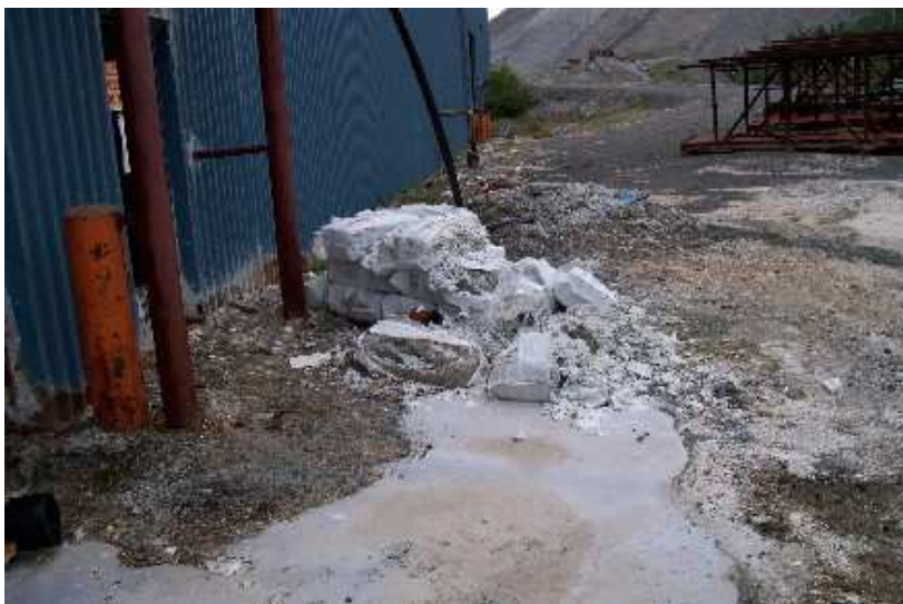
Photo 17: Damaged Bags of Asbestos Product – Southside of Wet Mill.
