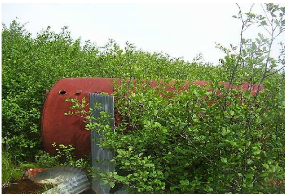
Photo 17. Discarded 10,000-Gallon UST. (Warehouse and Dock Area)
