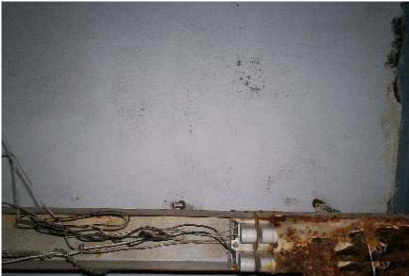
Photo 47: Light Fixture with no Florescent Light Ballast – Main Floor of Mine Dry.
