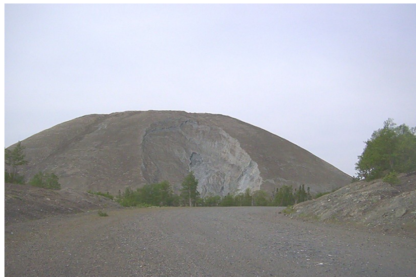
Photo 2: Slump at Eastside of the Tailings Pile.
