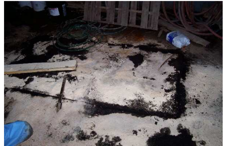
Photo 4. Possible UST inside of the Former E&R Building. (Former Northco Property)
