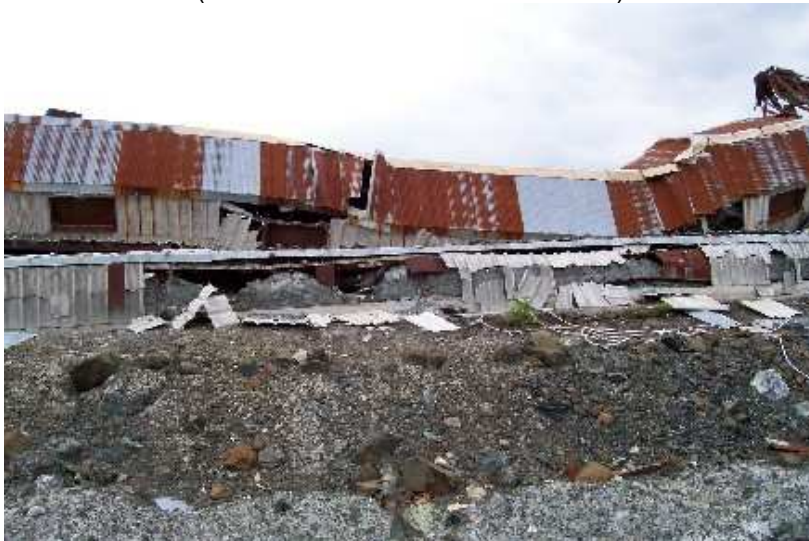
Photo 15: Exposed Friable Asbestos – Dry Rock Storage Facility and Associated Conveyor.
