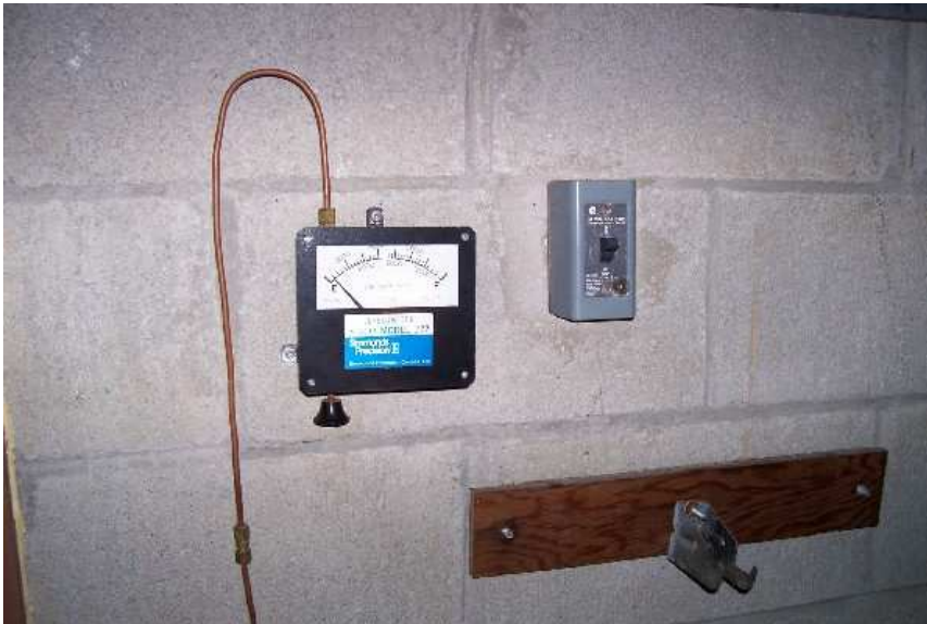
Photo 27: Fuel Levelometer in Boiler Room of Mine Dry. (Fuel Capacity of 13,367 Litres)
