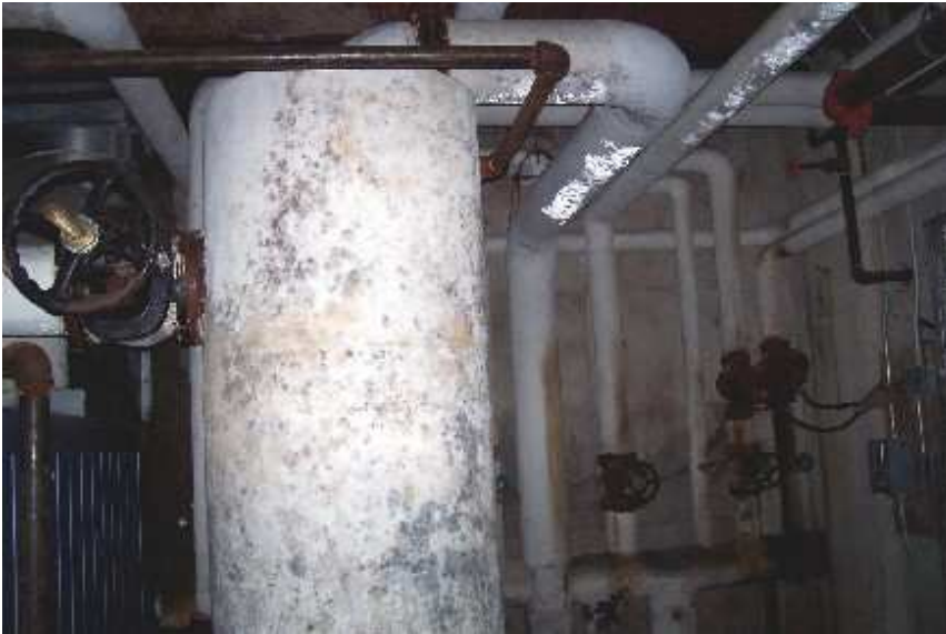
Photo 21: Boiler and Pipe Insulation – Boiler Room of Mine Dry. (Note Mold Growth)
