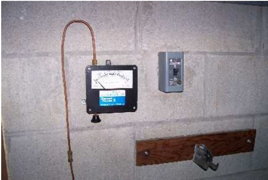
Photo 5: Fuel Tank Levelometer – Boiler Room of Mine Dry. (Former Northco Property)
