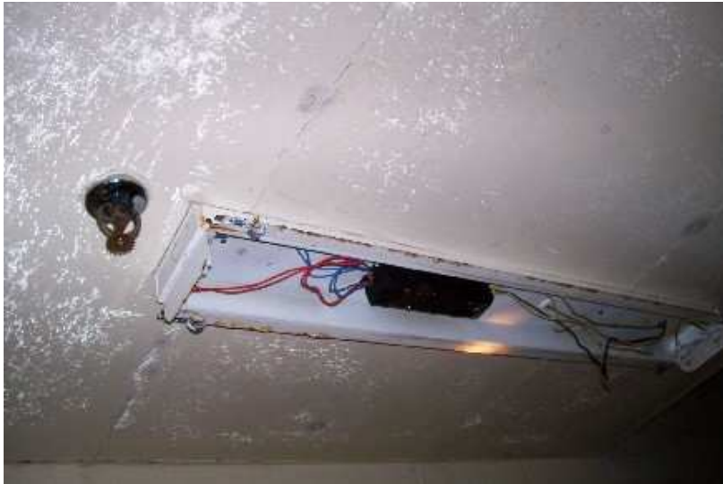
Photo 45: Florescent Light Ballast – Main Floor of Mine Dry.
