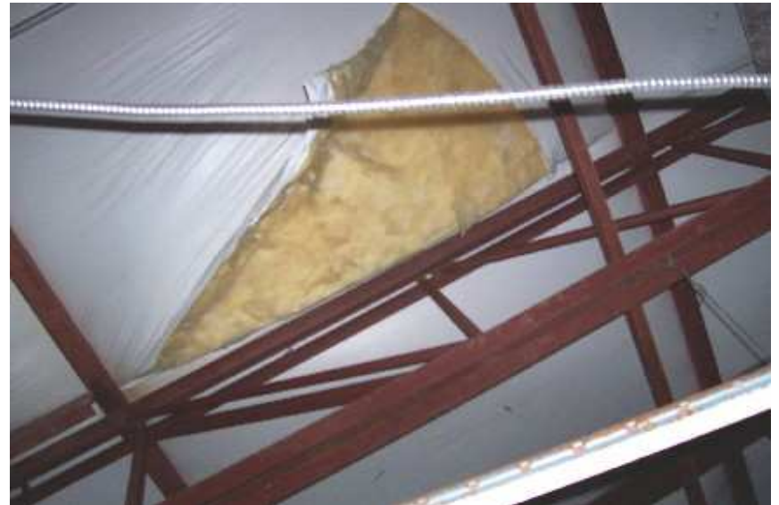
Photo 28: Fiberglass Insulation – Main Floor of Mine Dry.
