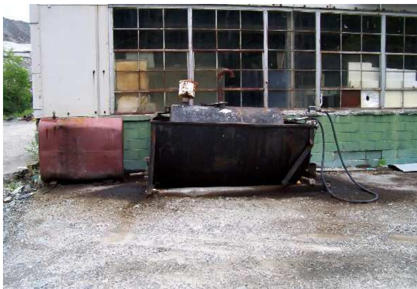
Photo 7: 1,000-Gallon and 200-Gallon Diesel Fuel ASTs – Adjacent Former E&R Building. (Note Staining on Asphalt)
