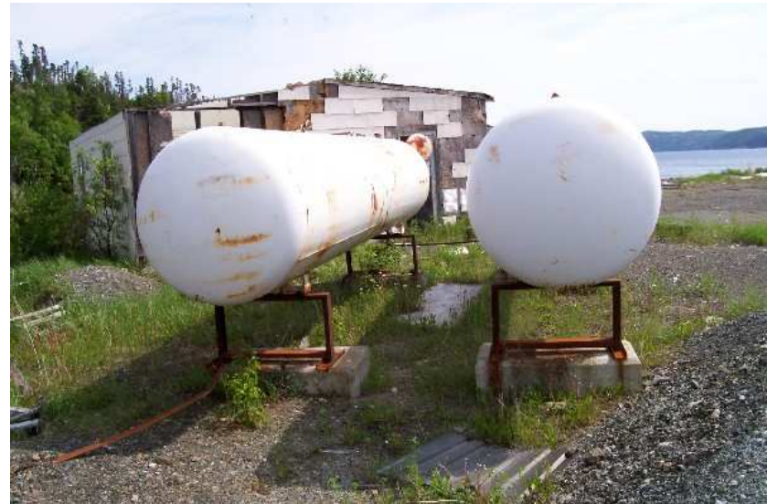
Photo 4. Two Propane ASTs located West of Warehouse. (Note the Former Lunchroom in Background)
