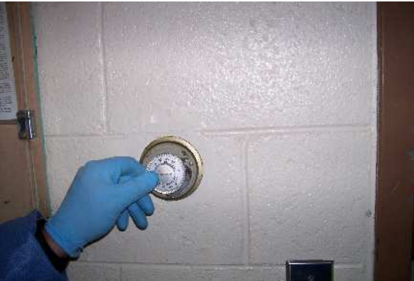
Photo 23: Typical Mercury Containing Thermostat – Main Floor of Mine Dry.
