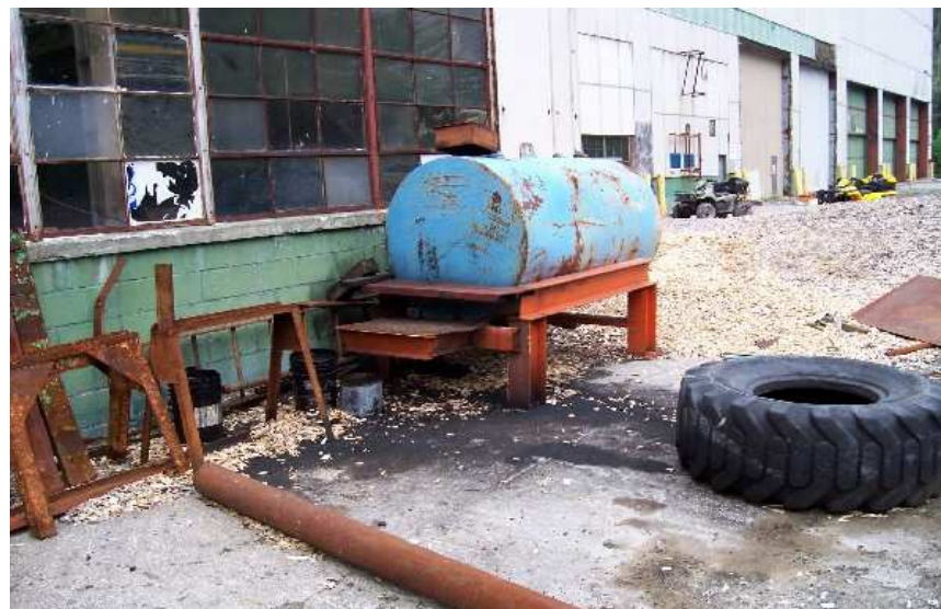
Photo 6: 1,000-Gallon Waste Oil AST – Adjacent Former E&R Building. (Note Staining on Asphalt)
