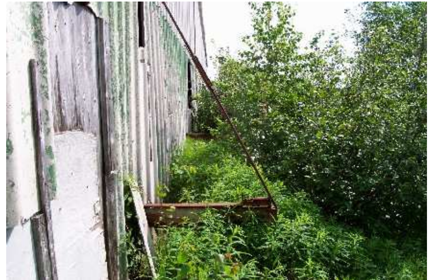
Photo 10: Metals Hangers Along Southeast Side of Warehouse. (Previous Location of Bunker C Pipeline)
