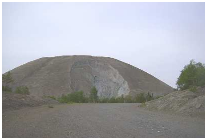
Photo 12: Slump – Tailings Pile.
