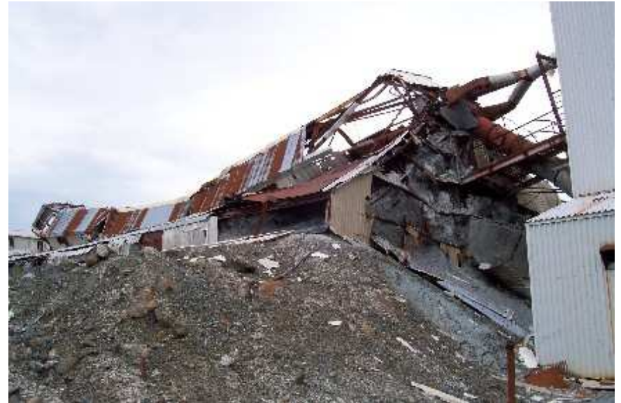
Photo 14: Exposed Friable Asbestos – Dry Rock Storage Facility.
