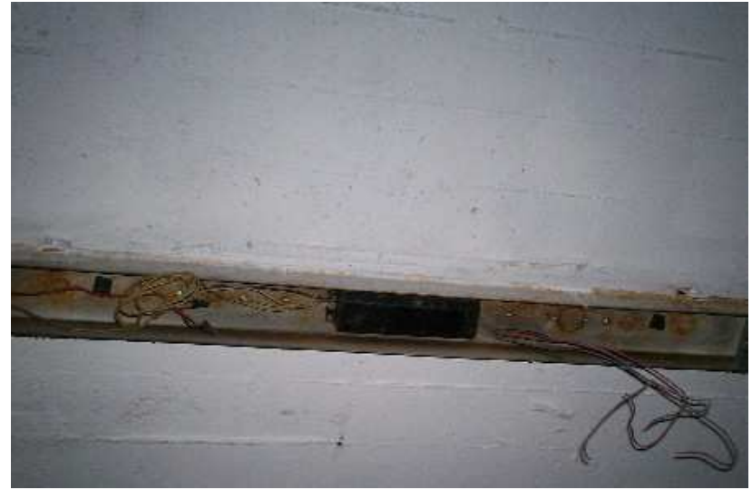
Photo 46: Florescent Light Ballast – Main Floor of Mine Dry.
