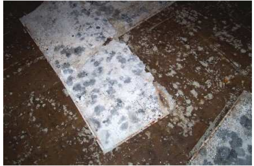
Photo 22: Mold Growth on Ceiling Tile – Basement of Mine Dry.
